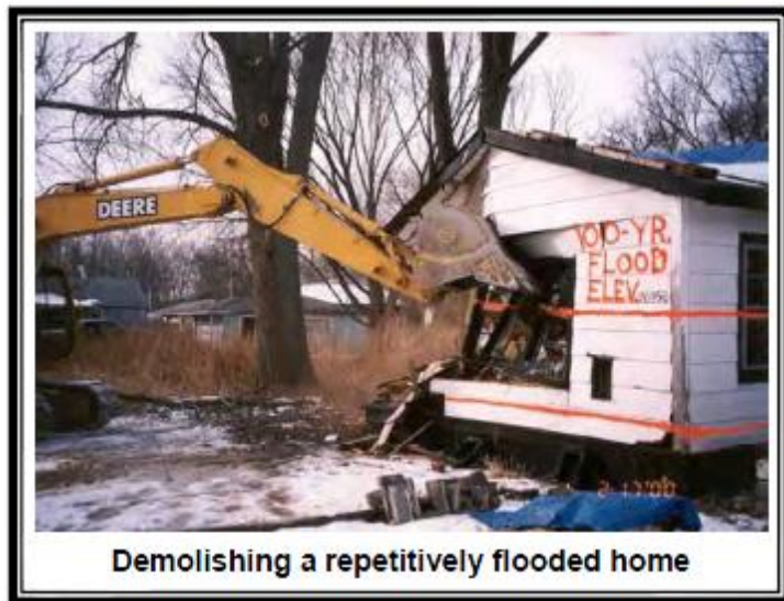
Figure C-5 Demolition of Flooded Home
