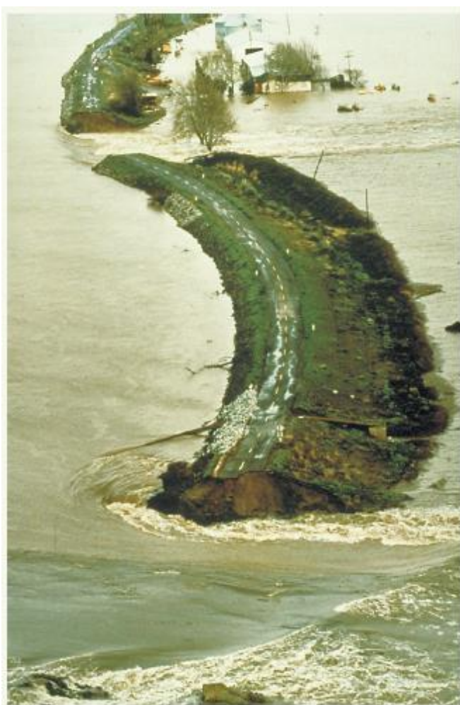
Figure 4-49 1986 Tyler Island Levee Breach
