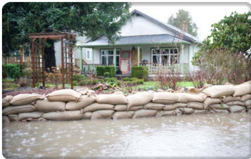
FIGURE 8 Temporary Flood Barrier
