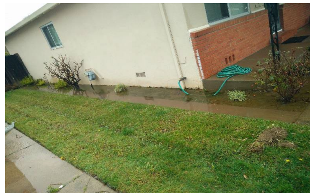
FIGURE 31. PONDING CAUSED BY LANDSCAPING OBSTRUCTIONS
