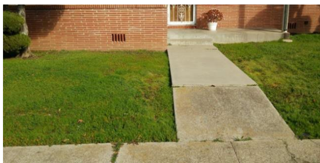
FIGURE 36. CRAWL SPACE UTILIZED AS A FLOODPROOFING MEASURE TO PREVENT FLOODING IN THE STRUCTURE
