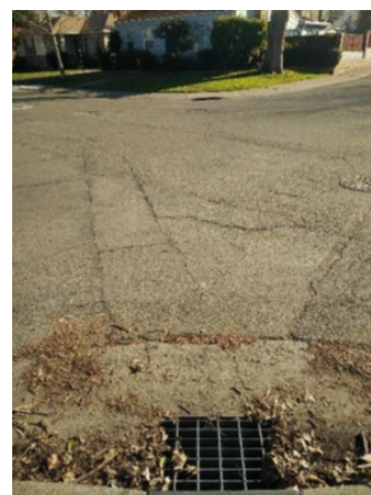
FIGURE 12. DEBRIS COLLECTING ON A STORM DRAIN AT THE CORNER OF 45TH AND C STREETS
