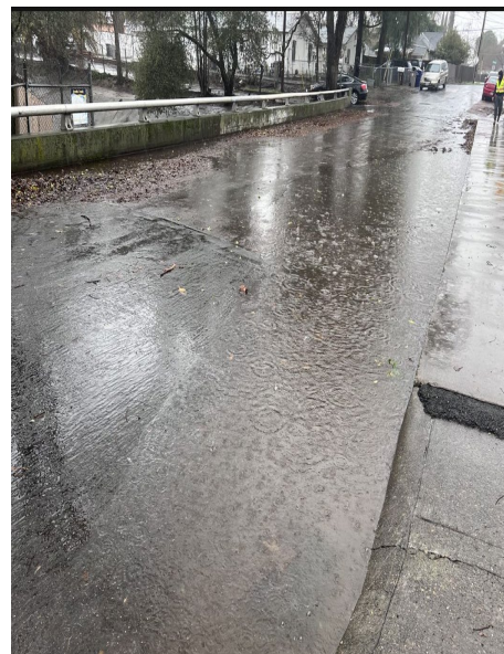
FIGURE 48. VERANO BRIDGE WATER PONDING
