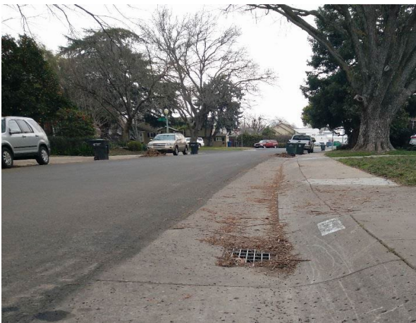
FIGURE 19. EXAMPLE OF DEBRIS IN THE STORM DRAIN. LEAF PILES ARE ALLOWED TO BE LEFT ON STREETS FOR CITY PICKUP AFTER CURBSIDE BINS ARE FULL; MANY TIMES, THESE LEAVES CAN CLOG THE STORM DRAIN
