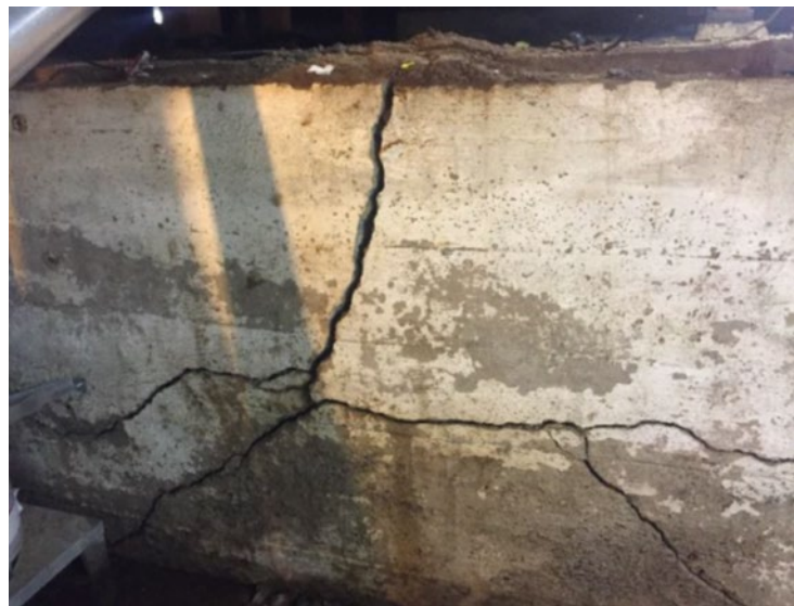
FIGURE 18. A FRACTURED BASEMENT WALL CAUSED BY HYDROSTATIC PRESSURE; CRACKS HAVE LED TO WATER SEEPING INTO THE BASEMENT
