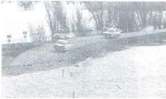
Figure 2.14. Flooding on Franklin Boulevard in 1964
