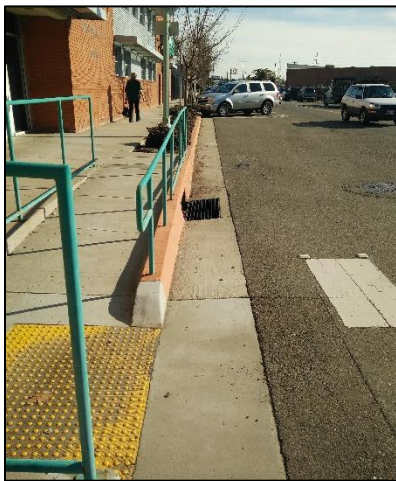
Improved drainage system project on Elvas Avenue that was completed in 2009.
