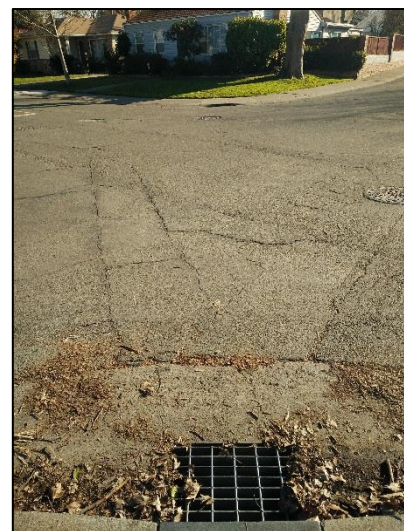
Right: Debris collecting on a storm drain at the corner of 45 th and C Streets.
