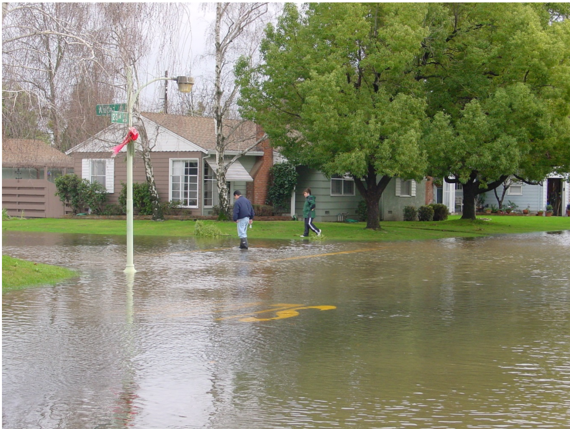
Figure 6.1. Flooding Caused by Internal Drainage Issues, Anita Avenue and 23 rd Street
