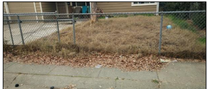
Debris obstructing the flow of water from exiting the property during storm events.
