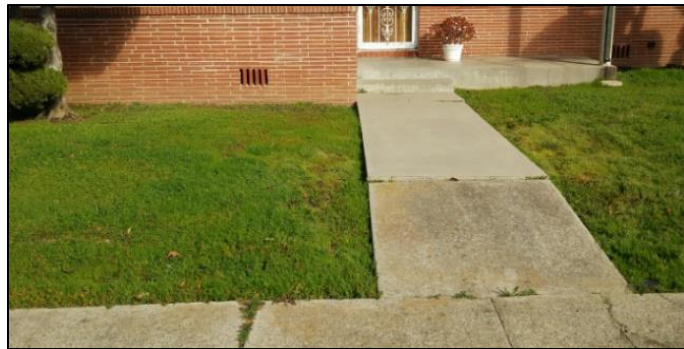
Crawlspace utilized as a floodproofing measure to prevent flooding in the structure.
