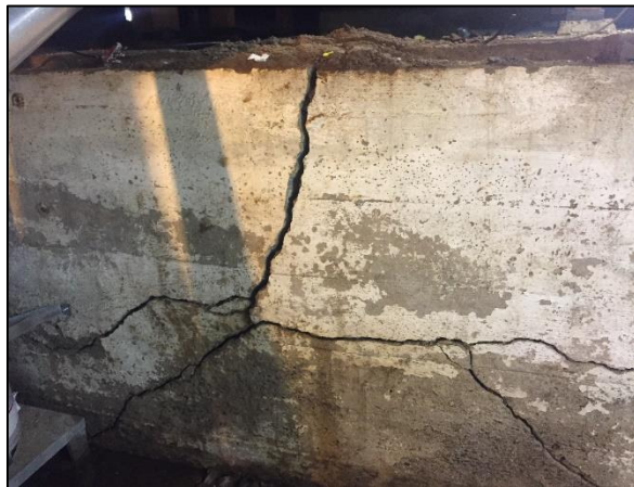
Left: On-site drainage added to aid in storm water drainage. Right: A fractured basement wall caused by hydrostatic pressure. The cracks have led to water seeping into the basement.
