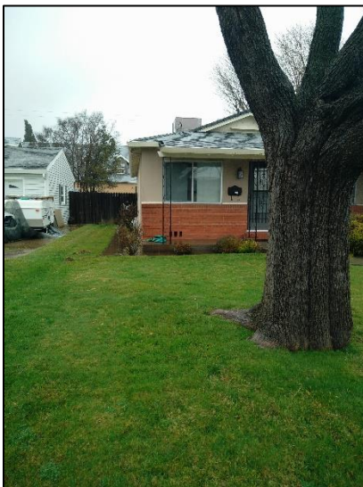
Structure built upon a crawlspace and HVAC unit is elevated as a flood proofing measures.
