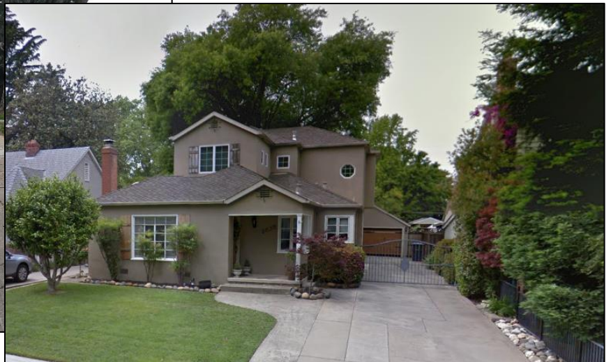
Example of a typical home in this area that wouldn't flood. Elevated on a crawlspace and the garage located in the back of the property. Some homes have basements.
