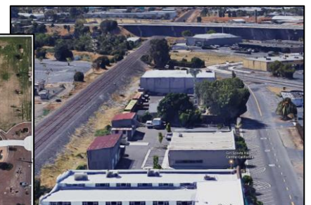
Overview of Area 4
