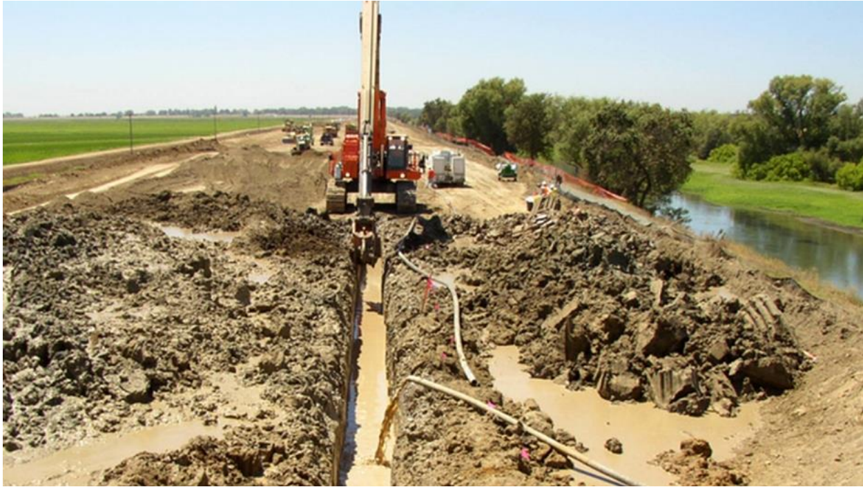
Figure 5.4. Natomas Levee Slurry Wall being constructed
