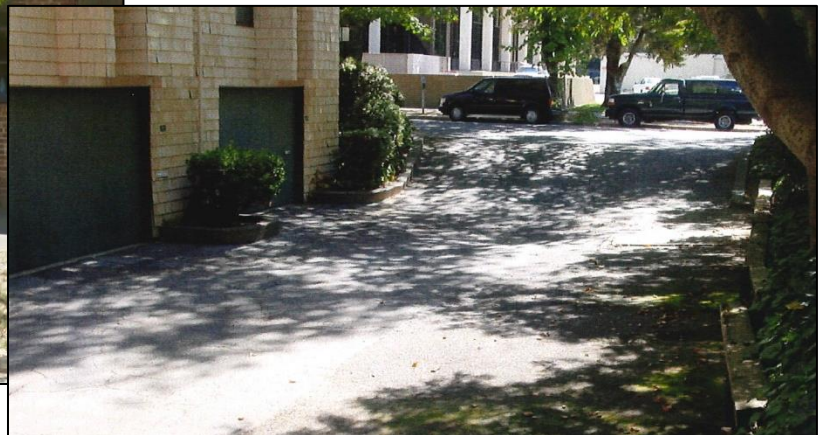
Garages are located below grade.
