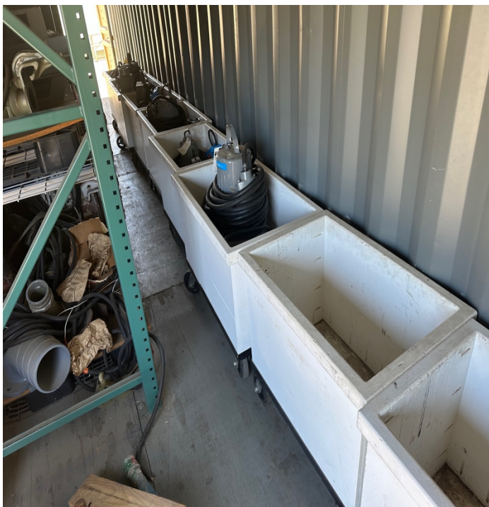
Task A (Photo A5): Inspection of City spare part inventory (view 1); management indicated some issues with timeliness getting some backup parts ordering affecting backup parts for system.
