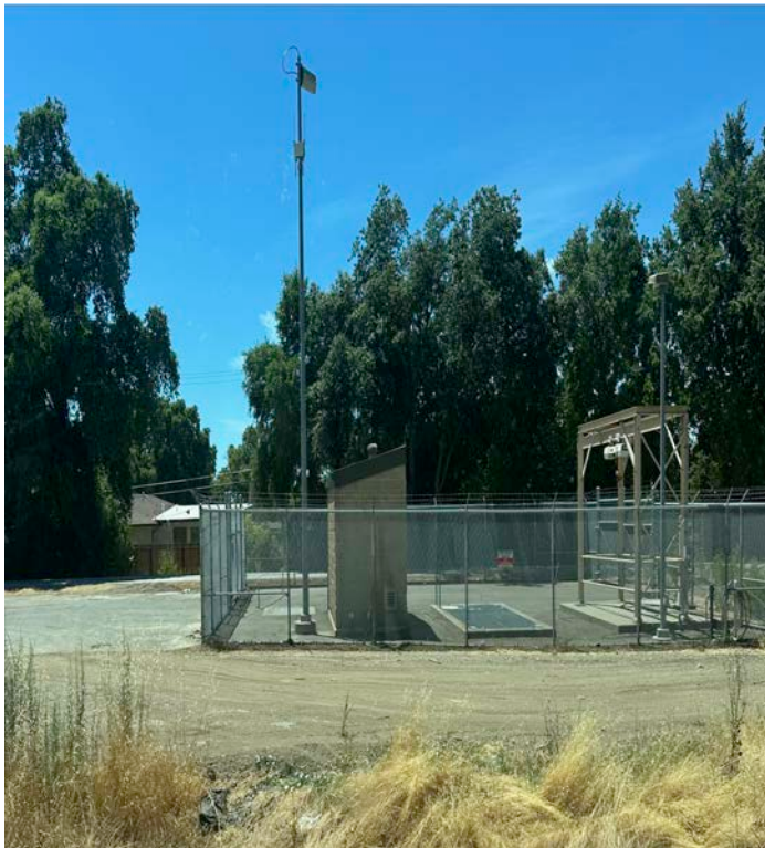
Task B (Photo B1): Inspection of Sump 21 pump station (view 1).
