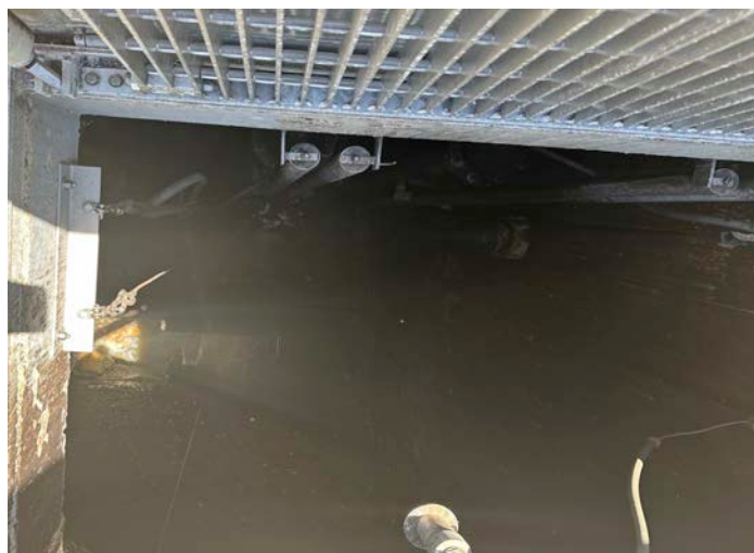
Task B (Photo B3): Inspection of pump station wet well; no significant corrosion, solids, or a grease mat buildup on top of flow observed.
