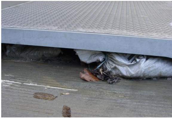
Avoid clogging inlets with gravel bags.
