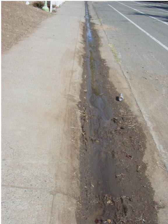
Construction sediment and debris should be swept as soon as possible.
