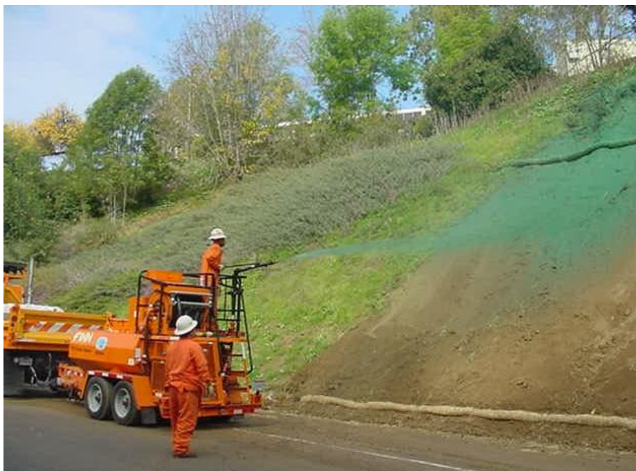
Green dye is often used to facilitate adequate and even coverage.
