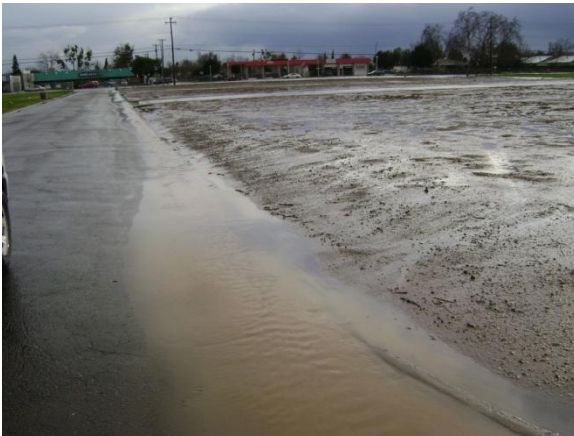
Significant erosion can occur when no soil binders (or perimeter controls) are provided.
