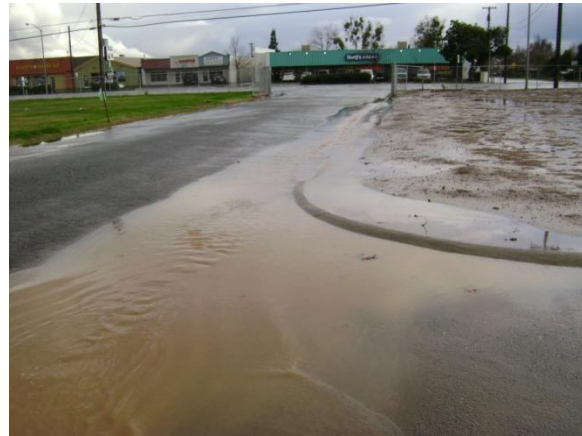
Significant erosion can occur when no soil binders (or perimeter controls) are provided.
