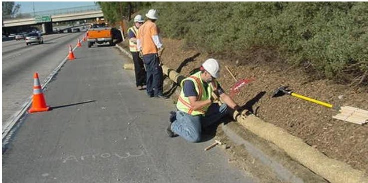
Wood stakes help secure fiber rolls.
