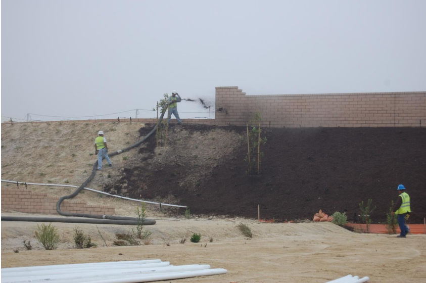
Mulching can be applied by hand or using pneumatic methods (as shown in this photo).
