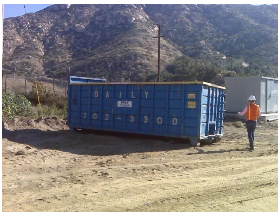
Although this large elevated trash container is easily accessible, it should also be covered or have secondary containment measures.
