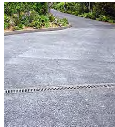
Pervious Driveway. Photo: Carrera Construction
