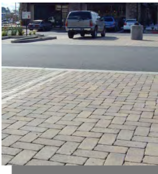
Porous Pavement at Fair Oaks Promenade, City of Folsom
