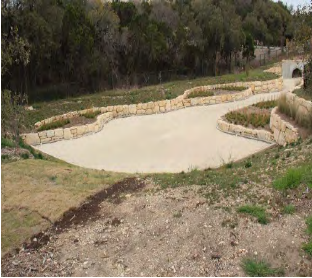
Figure A: Media Filter BMP Image County of San Diego LID Handbook BMP Image
