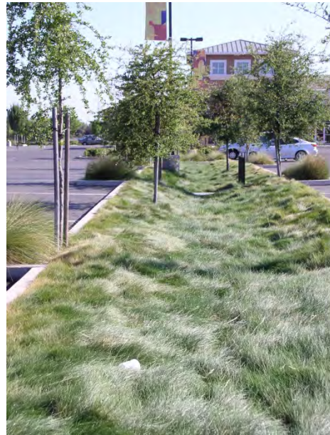
Vegetated swale, The City of Sacramento
