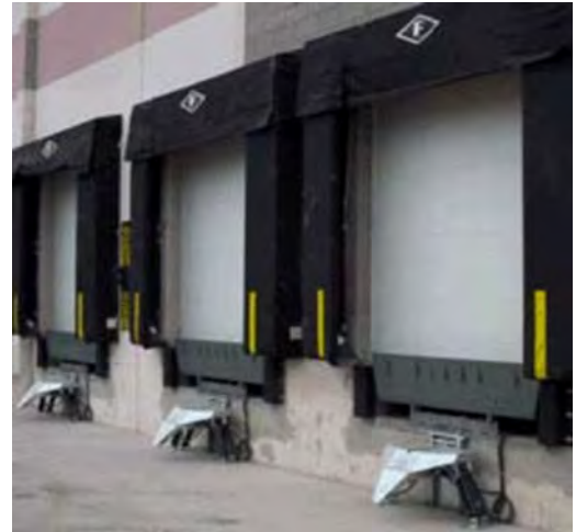
Delivery loading/unloading area. Photo source unknown
