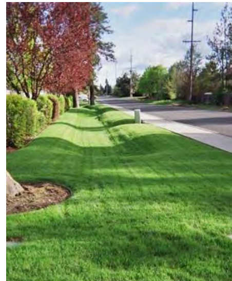
Roadside Swale. Photo: City of Spokane
