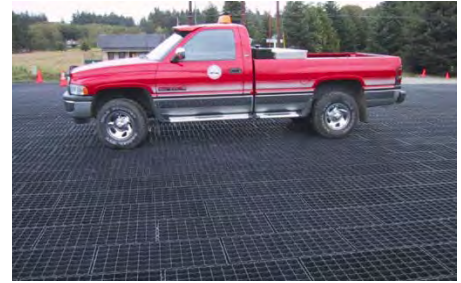
New installation of reinforced grass pavement. Photo: Puget Sound Action Team, WA
