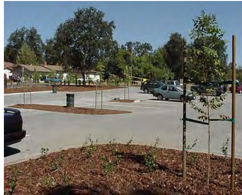
Pervious concrete parking lot; Bannister Park, Fair Oaks, CA. Photo: CNCPC and Fair Oaks Recreation and Parks District
