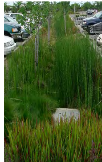
Alternative vegetation is encouraged but is subject to approval of local permitting agency. Parking lot swale at Elk Grove Marketplace, Elk Grove, California. Photo: CKB Environmental
