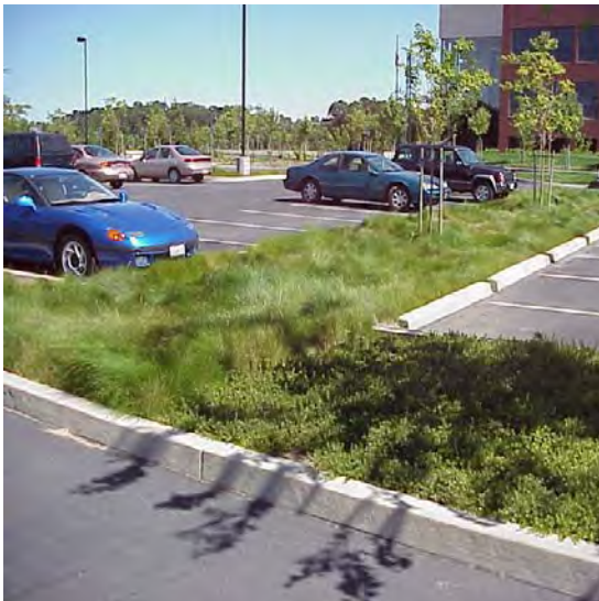
Vegetated Swale Planted with Native Clump Grasses (note that trees should be located outside of flowline), U.S. Farm Bureau, Sacramento. Photo: City of Sacramento.
