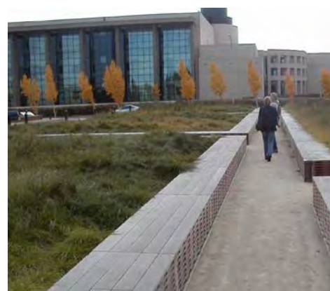
Pedestrian Walkway on Stanford University Parking Garage Green Roof, Palo Alto, California. Design by Rana Creek Living Architecture.
