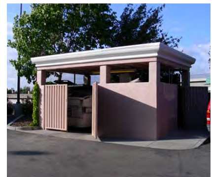
Covered Storage for Waste and Recycling Bins and Compactor, Pleasanton, California Photo: CKB Environmental
