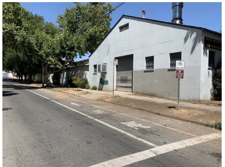
Northbound 28 th Street
