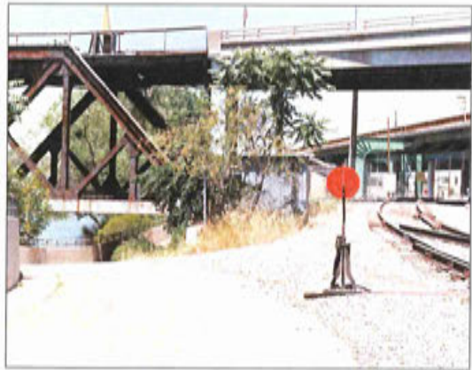
Resolving circulation conflicts as pedestrian and bike trails in Old Sacramento meet the excursion rail line at the "I" Street Bridge are critical for connecting the promenades on both sides of the River.
