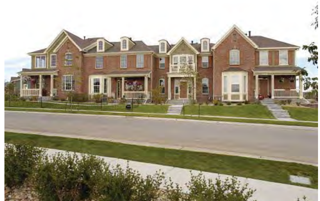
Broken roof pitches extending over porches, patios, or other similar features are encouraged.
