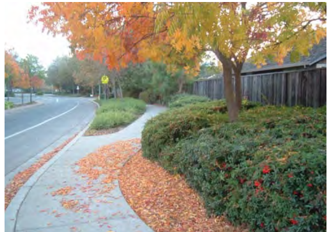
Residential collector with separated sidewalks
