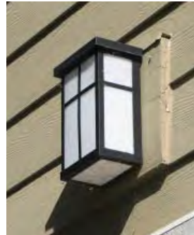
Wall-mounted light fixture
