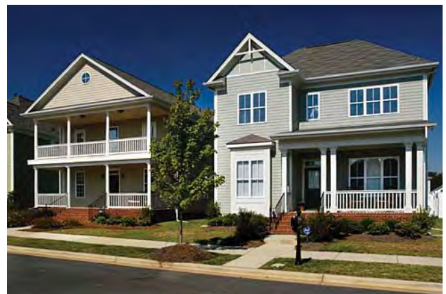
New construction may employ a variety of wood trim and siding profiles.
