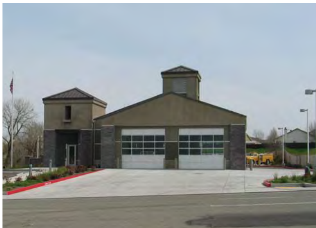
A site for a fire-station will be included within the Delta Shores Plan.
