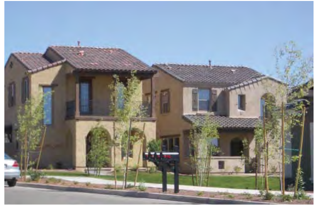
The architectural character, form, and massing should be varied through changes in roof form.
