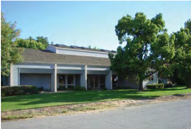
The Freeport community lacks curbs, gutters, and sidewalks.
