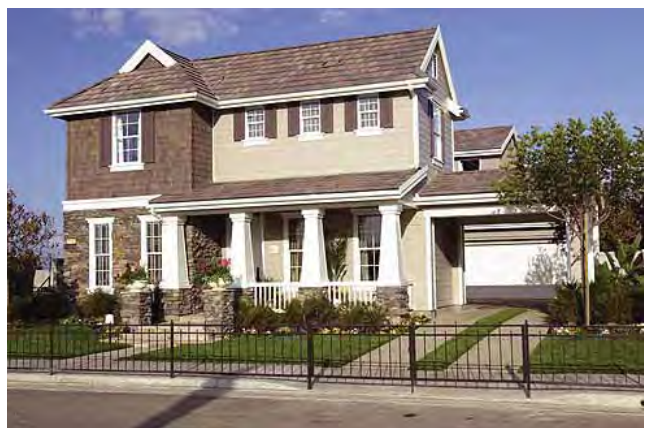
Homes with garages facing the street should offset garage door from front façade.
