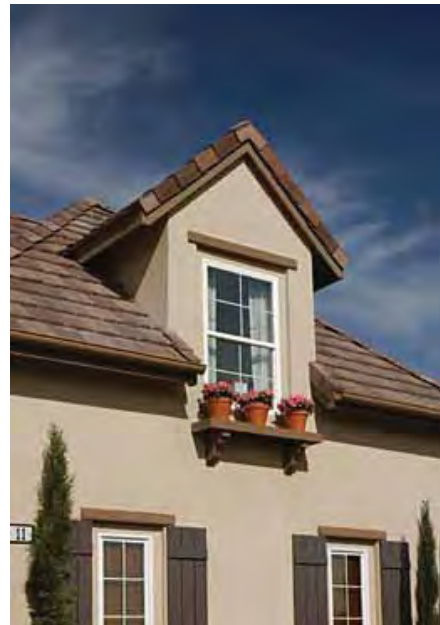
Dormer roof consistent with roof slope
