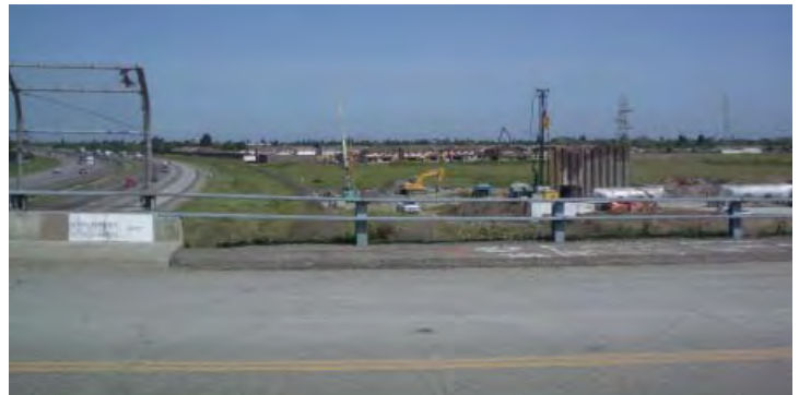
Stone Creek Road and construction on the Lower North West Interceptor
