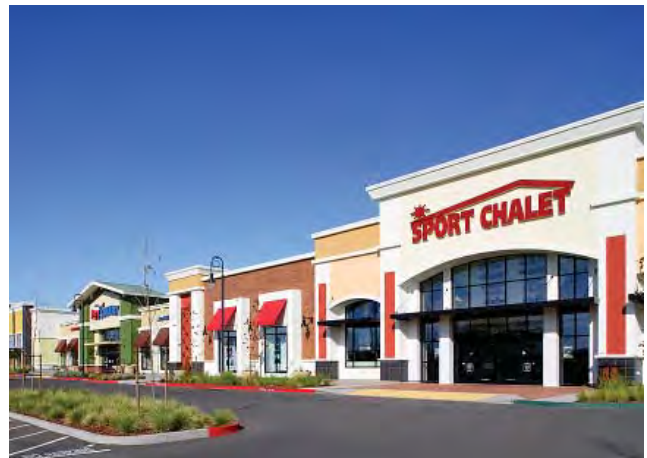
Building forms should be articulated to add interest and reduce the appearance of bulk and mass.
