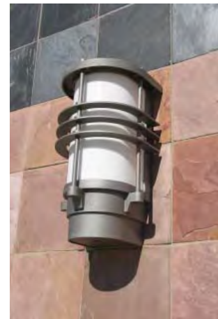
Wall-mounted light fixture
