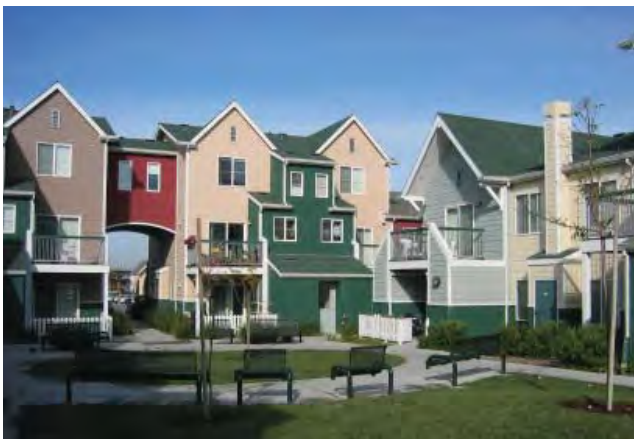
A private outdoor sitting area may be included within townhomes or apartments.
