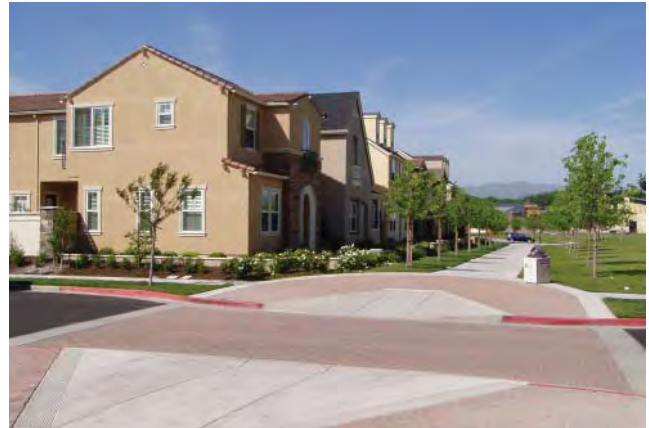
Wheelchair accessible sidewalks
