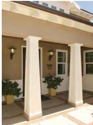
Traditional columns and brackets
