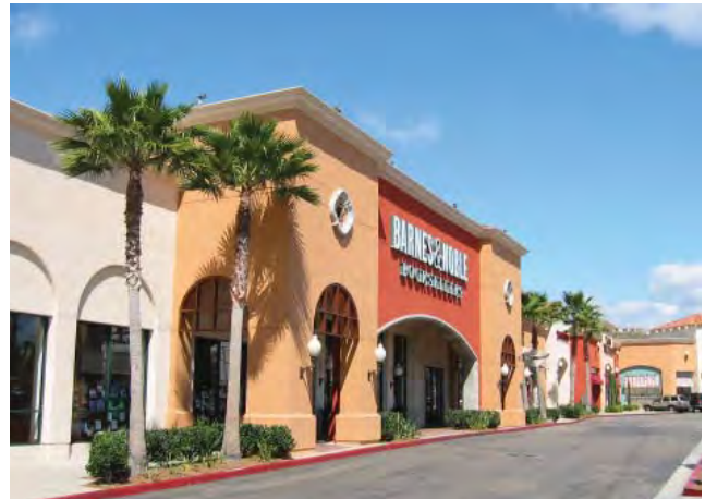
The building base should be visually anchored by use of articulated materials, architectural details or colors at the pedestrian level.
