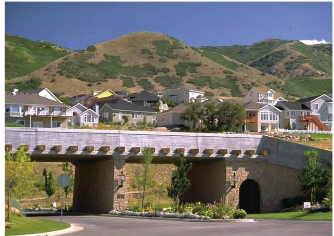
Bicycle and pedestrian bridge
