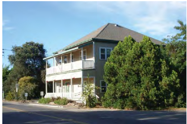
Typical porches and balconies on Freeport Boulevard
