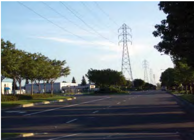
Typical photograph of electric towers within median.
