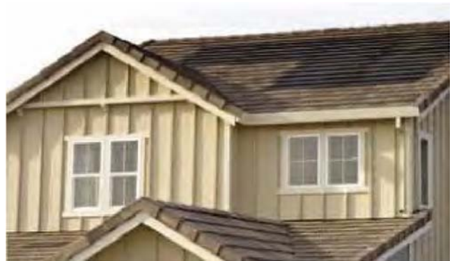
Building integrated photovoltaic panels.
