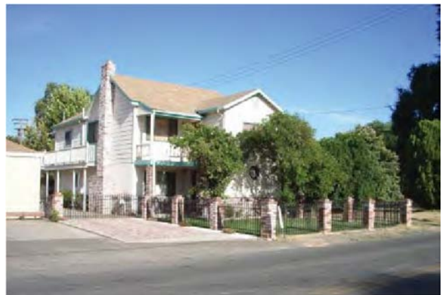
Freeport Boulevard residential building
