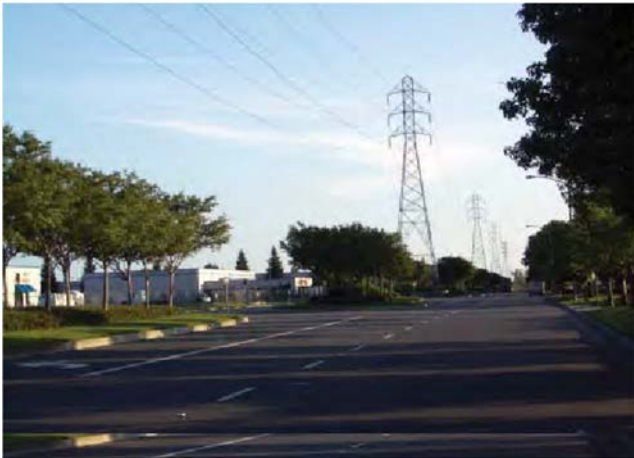
Typical photograph of electric towers within median.
