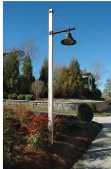
Landscaping around site lighting fixtures
