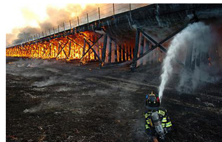
The Sacramento Fire Department responding to a fire emergency along a 300-foot stretch of an elevated Union Pacific railroad trestle.
