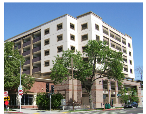
Multi-level parking structure.
