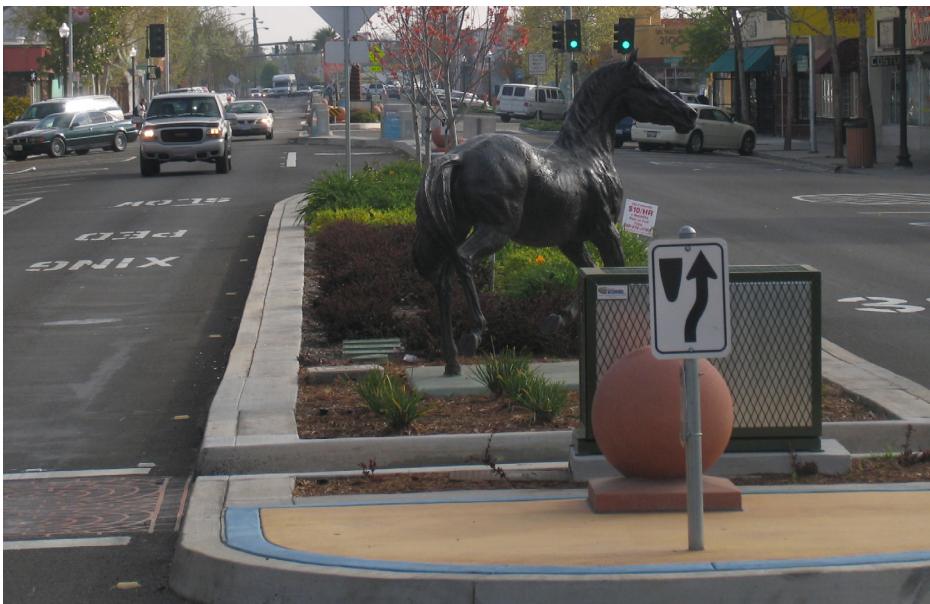
Safe pedestrian crossings, on-street parking, street trees, and landscaped medians on Del Paso Boulevard.
