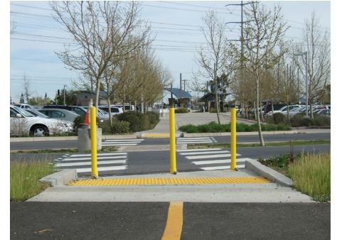
Meadowview Light Rail Station with pedestrianway and bikeway improvements.
