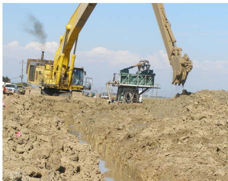
Improvements to levee infrastructure.
