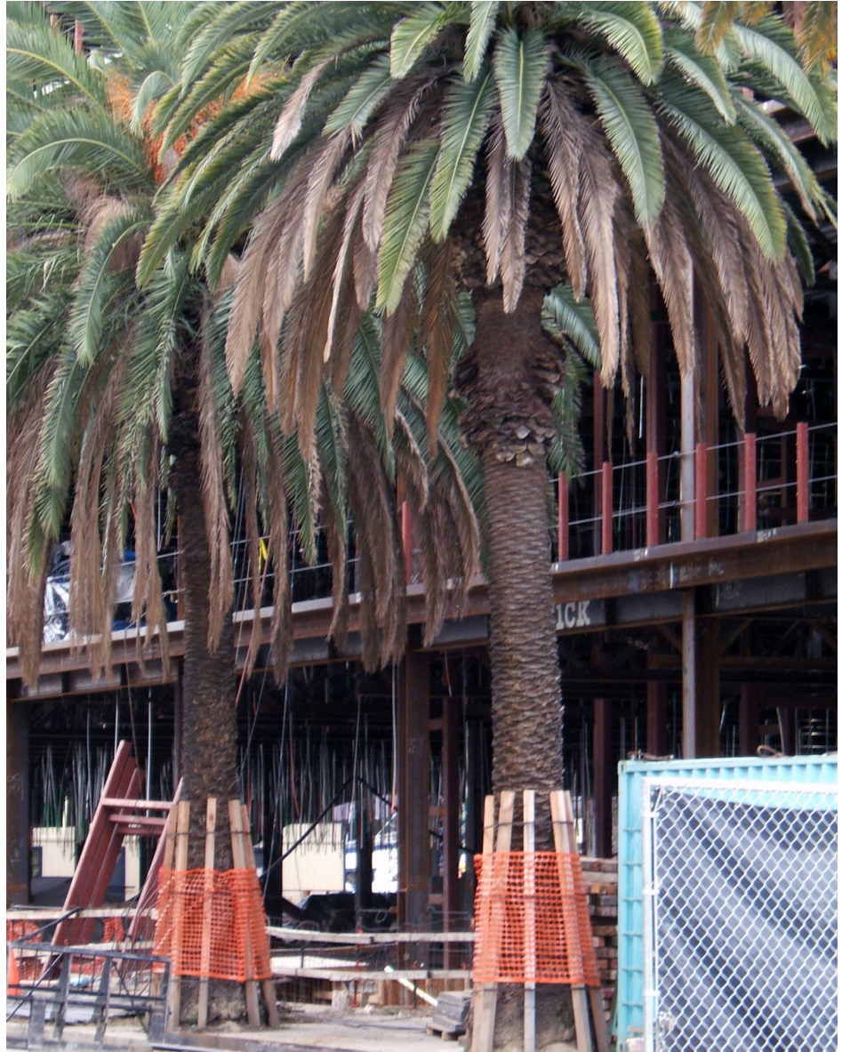
Preservation of existing palm trees in right-of-way adjacent to construction site.
