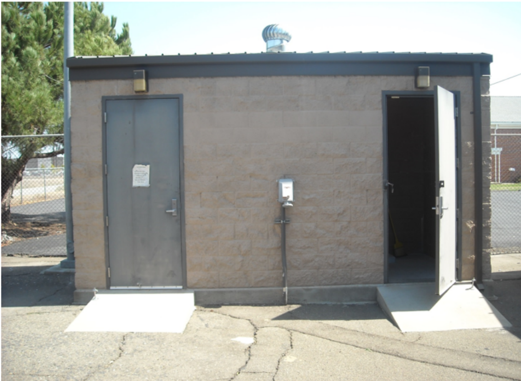
Photograph A. Sump 48 is typical of the pump stations that serve individual separated basins in the city's wastewater collection system. As shown in the photograph, Sump 48 is a separate dry pit/wet well configuration (one entrance for each), which is common for these pump stations.
