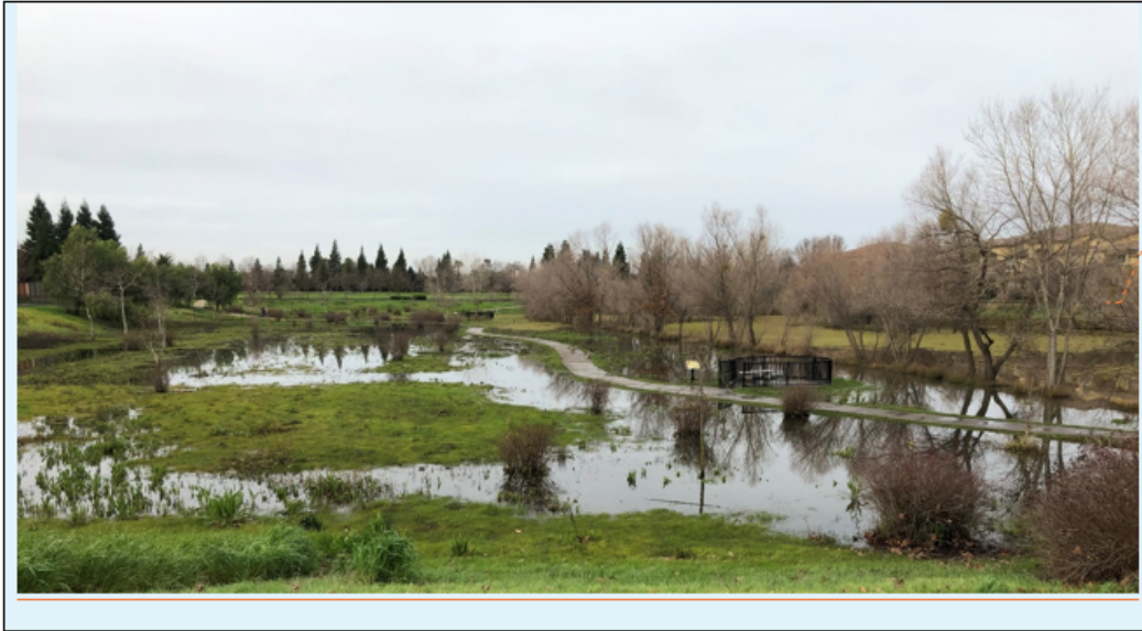
Photograph B. Basin 14 is located along Crest Drive. The wet portion of Basin 14 has a permanent water pool that provides stormwater quality treatment and wildlife habitat and includes a public path and benches in the bottom of the pool. When large storms occur, the paths and benches are inundated.
