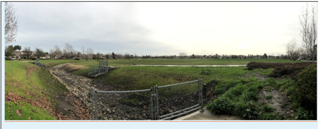
Photograph C. Basin 14 is located along Crest Drive. The dry portion of Basin 14 drains completely between storms, allowing use of the basin bottom for public access, sports fields, and other uses.
