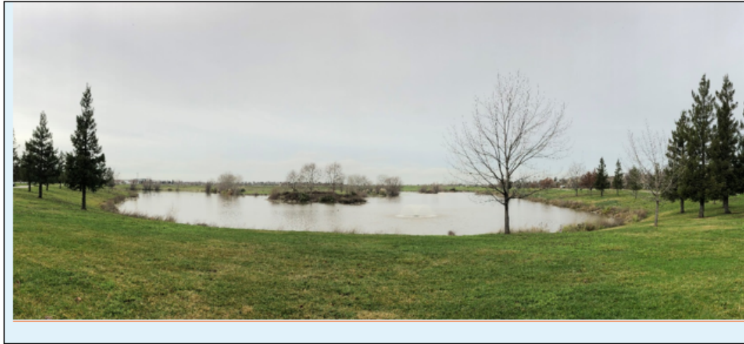
Photograph D. Basin 11 is located along Natomas Boulevard. Basin 11 has a permanent water pool. This basin provides flood control and stormwater quality treatment as well as wildlife habitat and a public path around the edges of the basin.
