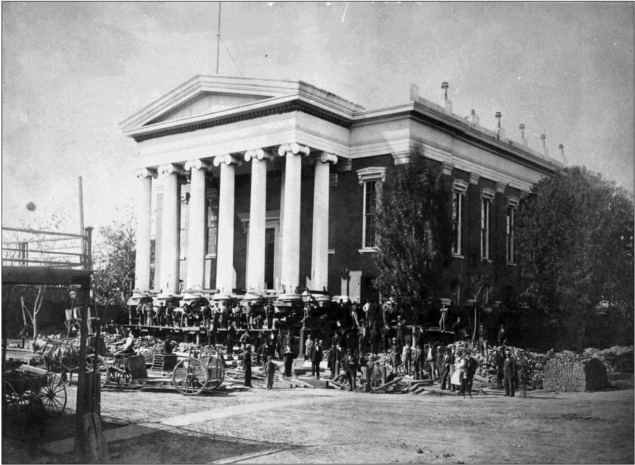
Figure 16. To avoid floodwaters, many buildings in Sacramento were raised in the 1860s and '70s. Pictured is the Sacramento County Courthouse being raised with jacks. [Center for Sacramento History, California State Library Collection, 1968/110/238].
