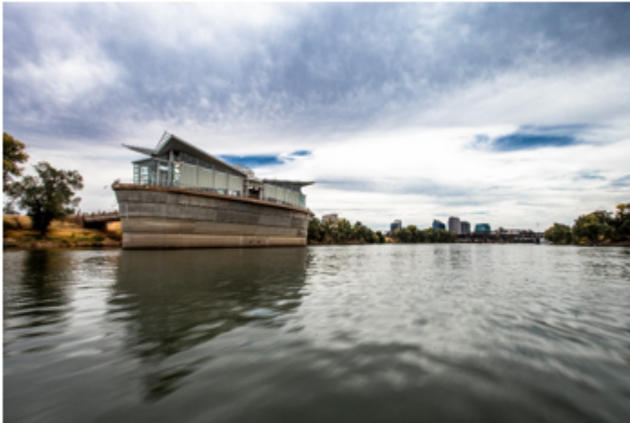
Photograph H. Sacramento River Water Treatment Plant Intake Facility
