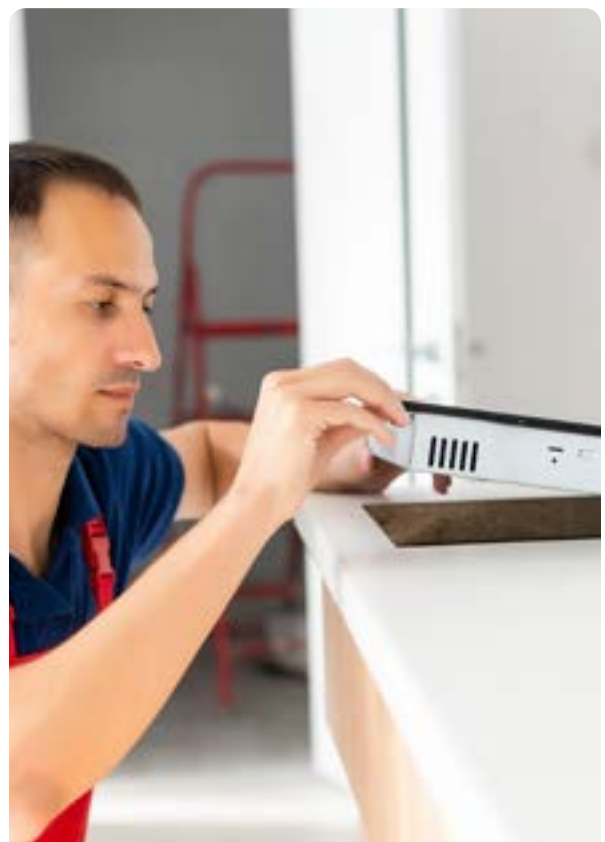
Induction Stove Installation
