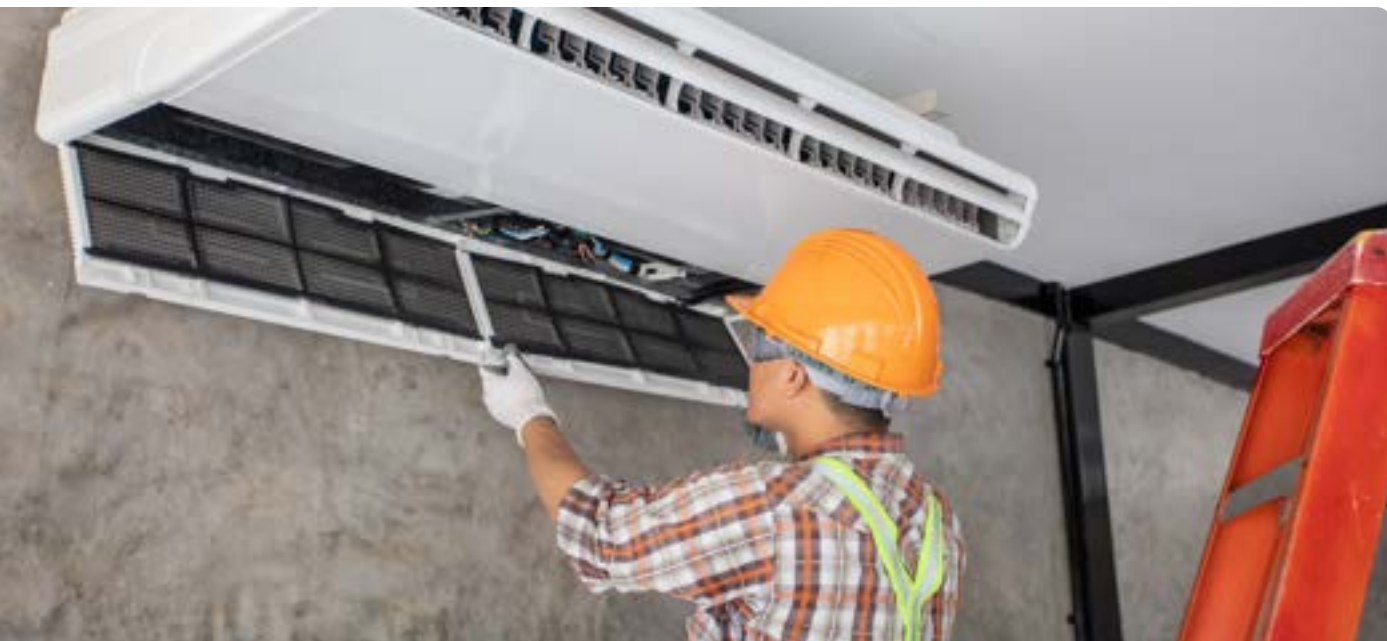
Electric Heat Pump HVAC Unit Installation
