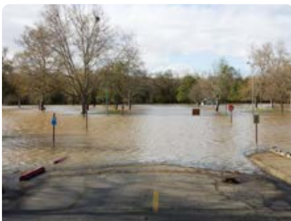
Flooded Sacramento Street
