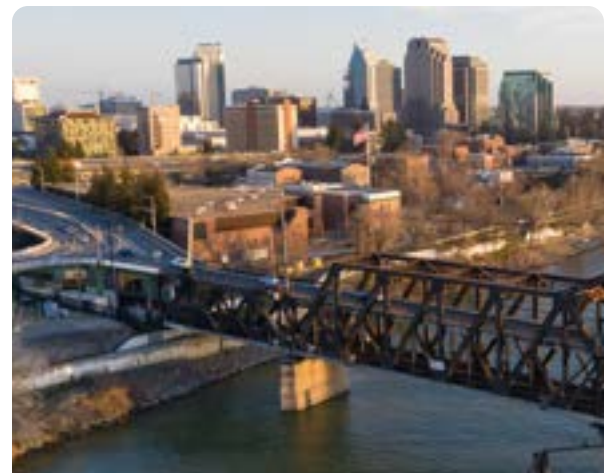
I Street Bridge and Downtown Sacramento
