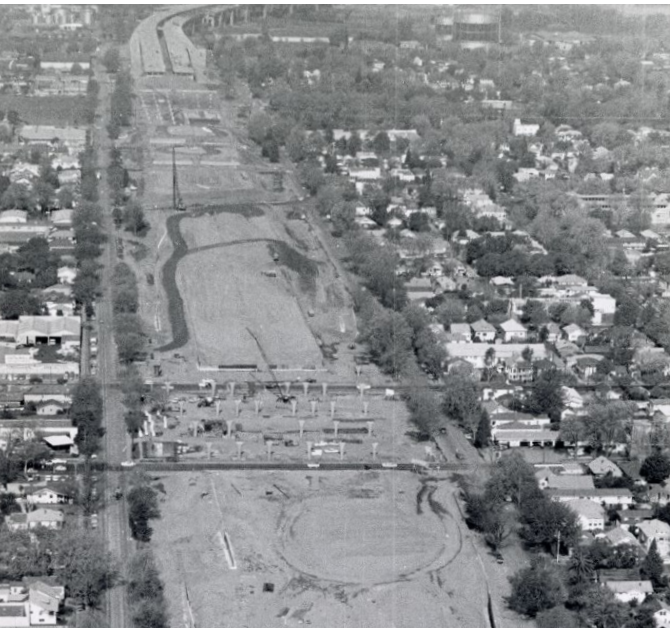
Capital City Freeway construction circa 1966.
