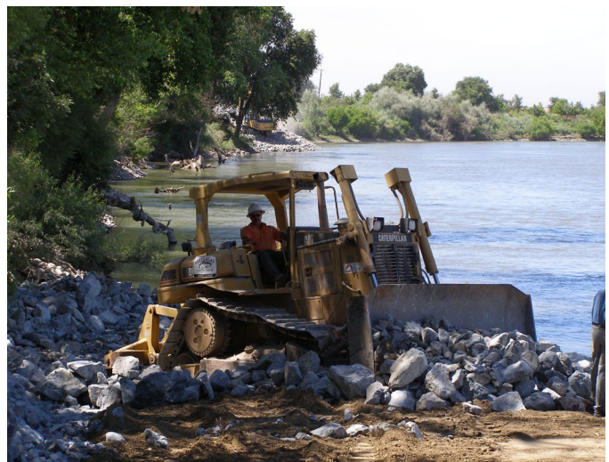
Replacing old levees is part of the flood protection plan.
