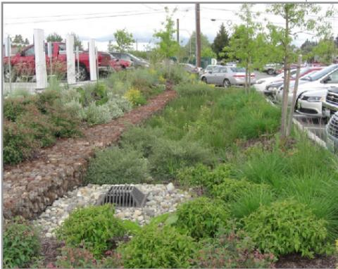
*Vegetated swales and filter strips effectively integrated with tree shading*
