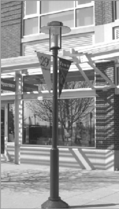
*Pedestrian pole lighting with a solid top eliminates light spillover and glare*
