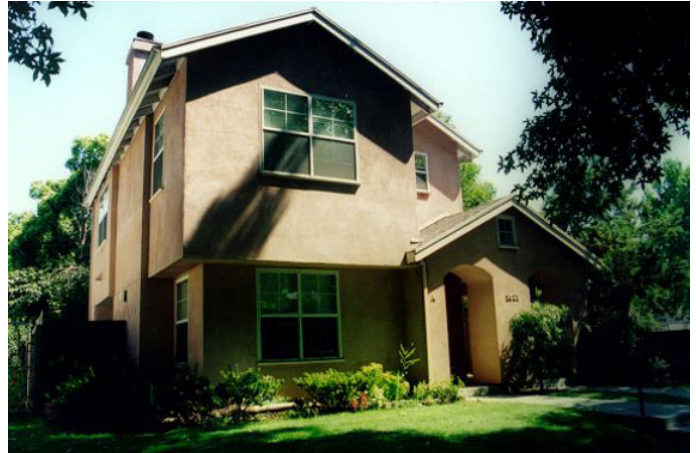
Figure 3-58. 1521 V Street. When plaster is used, smooth plaster texture is most compatible in the Central City.
