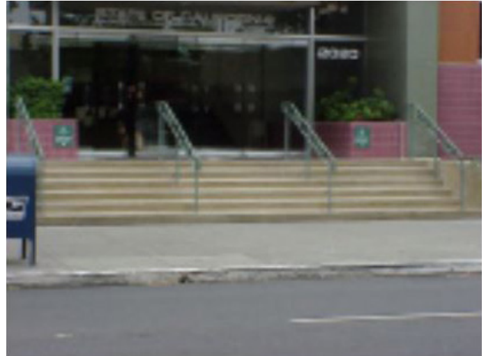
Figure 3.57. State EPA Building, L Street
