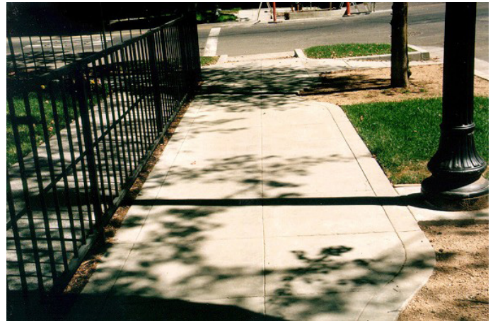
Figure 3-29. 27th & H. new sidewalk improvements should match the historic patterns.
