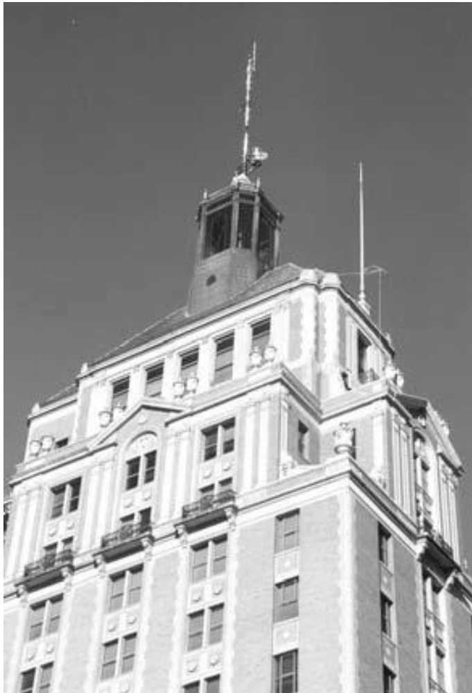
Figure 3-36. 921 11th Street. The Elks Building has a very powerful, uniquely articulated top.
