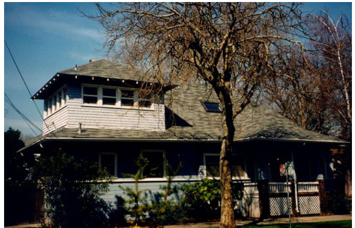
Figure 3-70. 2550 O Street. A second floor addition that is relatively consistent with the character of the original structure.
