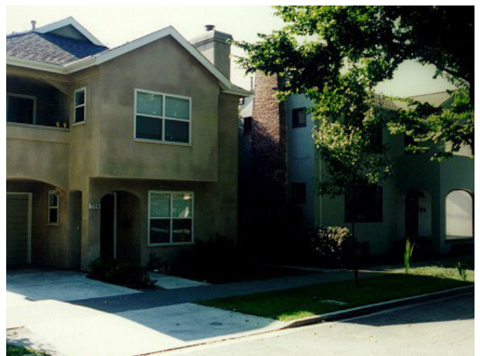
Figure 3-43. 703-705 26th Street. The structure on the left was built in the 1990s and utilized the plaster arch, porch, roof slope, and window patterns of the adjacent, much earlier, structure.
