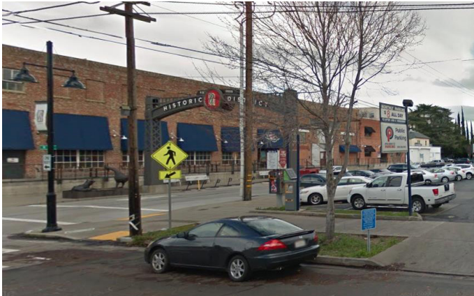
Figure 6-32. R Street at 10th. Sector A: Historic Industrial Sector A has a significant concentration of historic brick warehouse buildings and industrial uses. This western most segment features the strongest industrial character of the R Street project area. The traditional sharing of the roadway between pedestrians, bicyclists, and automobiles is most prominent in this area. Development of new buildings and streetscape elements provide a unique opportunity to maintain and strengthen the unique historic fabric of R Street. Image Credit: Google Maps
