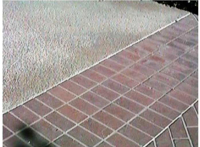
Figure 3-28. Brick on Concrete Paving.
