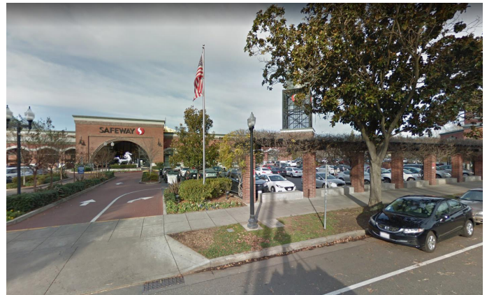
Figure 6-35. R-Street Market at 19th. This sector includes the largest inventory of boarded up and underutilized buildings, vacant open lots, and underused roadways along R Street. This contrasts with the recently built and well used "R Street Market." There is a tremendous opportunity to develop animated multi-use open and built spaces that will connect to this key anchor development and capitalize on its synergy with the east end of the Corridor. Image Credit: Google Maps
