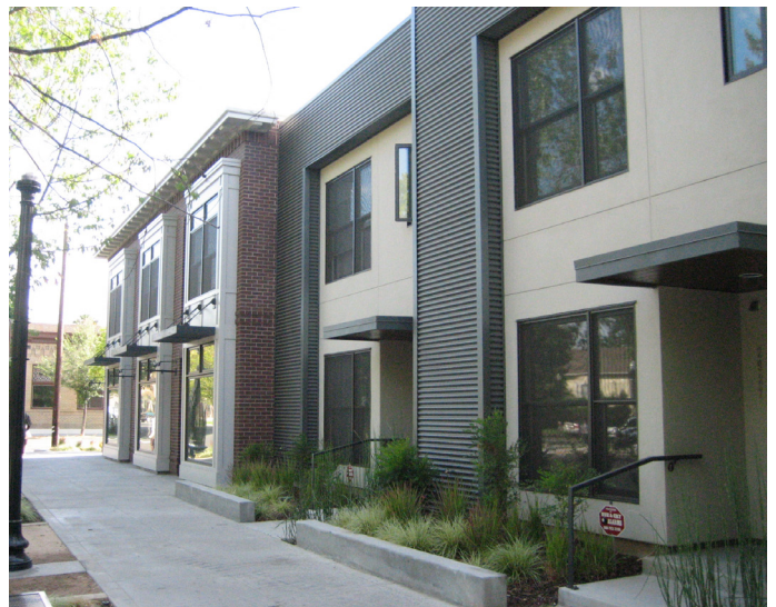
Figure 3-27. Planters with a raised curb, planted with ground cover and low shrubs
