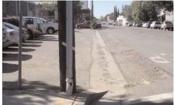
Figure 6-139. Vee gutters maintain the shared roadway concept on R Street.
