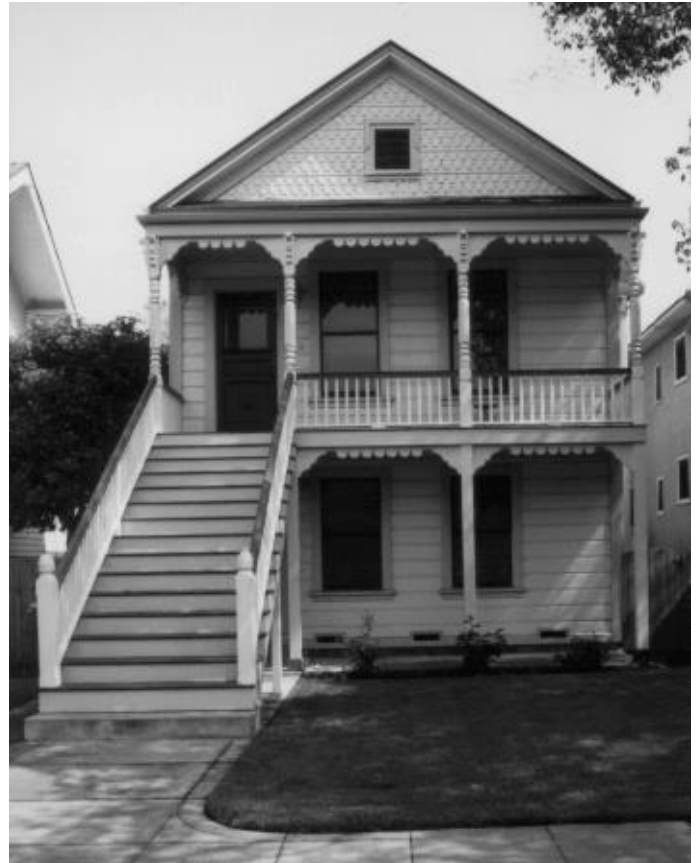
Figure 4-7. 2609 P Street. A typical Victorian workman's home.
