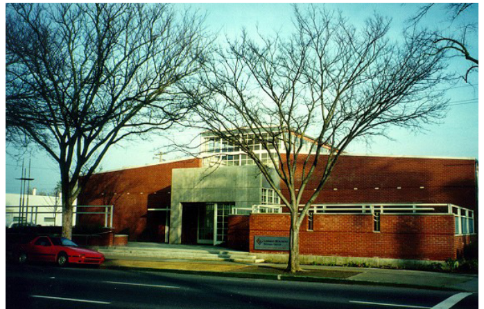
Figure 6-21. 19th and T. Parking should be oriented to the interior side and, where appropriate, to the rear of lots, as done in this renovation project
