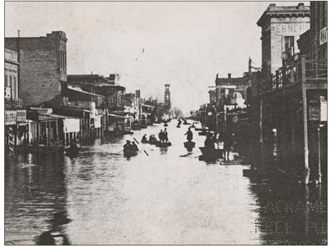
Flood damage in 1861 along K Street near Front Street
