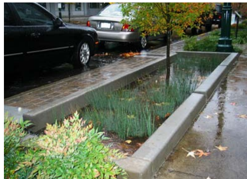
Integration of stormwater management features into street design can provide multiple benefits.
