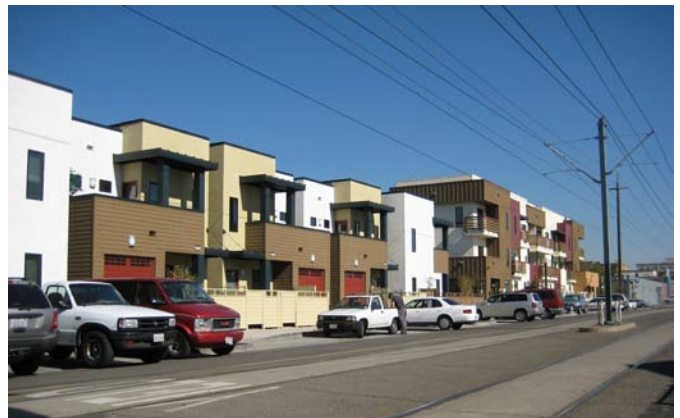
R Street at 25th medium density residential in-fill project.
