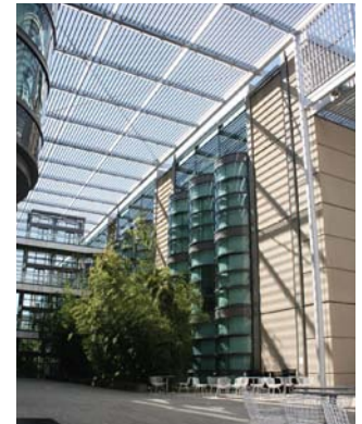
Figure 2. Giant sun-control canopy covering a the courtyard of a science building on the Stanford University campus.
