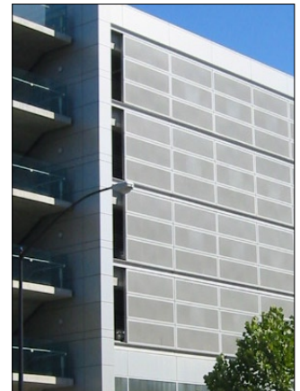
Figures 11 and 12. Parking structure at City Hall in San Jose, CA, uses horizontal metal louvers (left) and perforated metal panels (right) to control the glare produced by night lighting.
