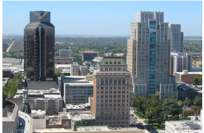
Figure 1. View of the River District, from the top of the Empire Building, looking west. These buildings employ a variety of stepback strategies, ranging from stepbacks only at the top to frequent stepbacks applied at various stages of as the buildings rise.
