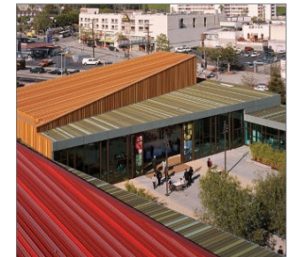
Figure 6. Metal wall and roof panels
