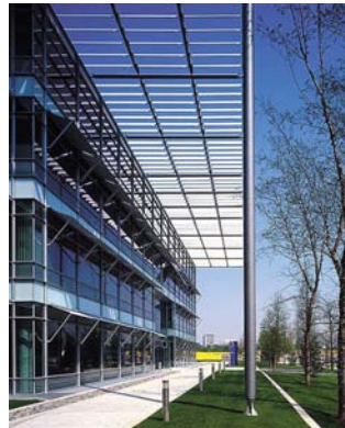
Figure 1. Giant canopy applied to a commercial office building, Chiswick Park, London, UK.
