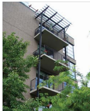
Figure 4. Stacked balconies on an apartment building
