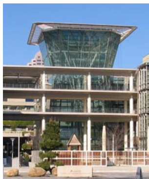
Figure 4. The CalPERS Building, Sacramento, CA. The building regulates air ventilation by channelling warm air up and out through the glass atrium.
