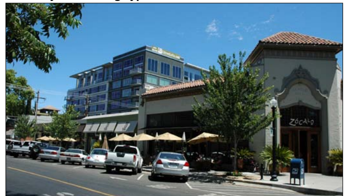
Figure 3: A variety of scale and form in a single block, as seen here at 18th and Capitol Streets, provides diversity of retail and living opportunities while retaining original historic resources.
