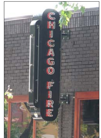
Figure 3. New blade sign with classic exposed neon further defines building details.
