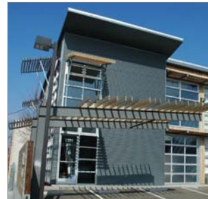
Figure 5. Industrial metal siding
