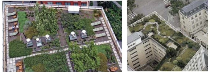
Figures 1 and 2. Green roofs can also be used as open space, can facilitate stormwater management, and reduce energy consumption by keeping a building cooler.
