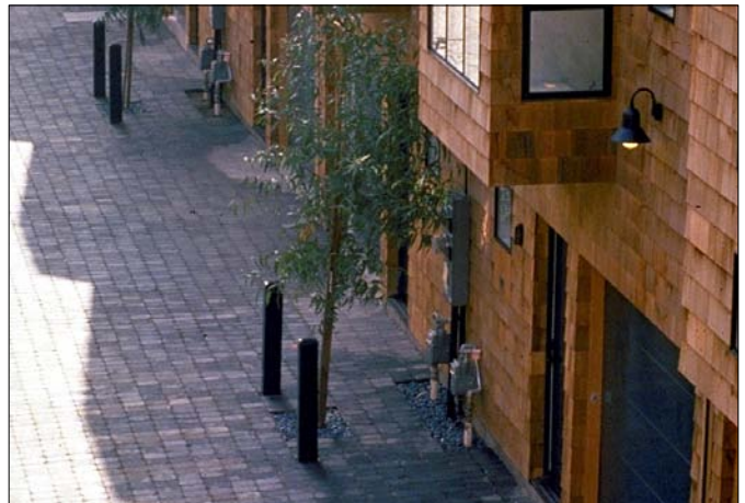
Figure 2: Utilities connections should be carefully located and integrated into the rhythm of the design.
