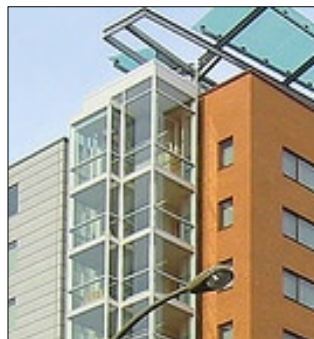
Figure 5. Rooftops and Mechanical Penthouse Enclosures
