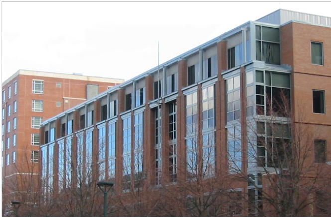
Figure 2. This university building in Cambridge, MA, has a repeating double window bay module which sets a rhythm across the facade, which is then interrupted by special conditions at the corner and above the entry.
