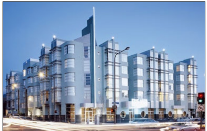
Figure 6. Lighting needs to be appropriate to a building's use and location. It should be integrated into the facade design, as seen here in the Fine Arts building along Shattuck Avenue in Berkeley.
