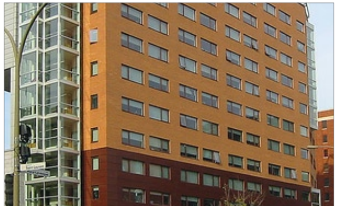
Figure 5. The windows in this mid-rise building provide operable window systems, which in the River District would be advantageous to collect delta breezes for occupant comfort.
