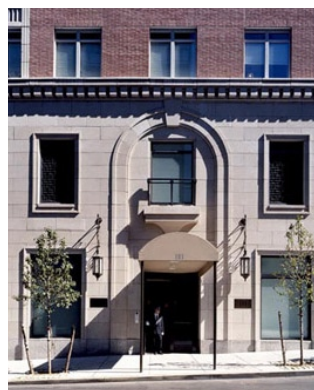
Figure 1. Entrance canopy to a residential apartment building on a downtown street.
