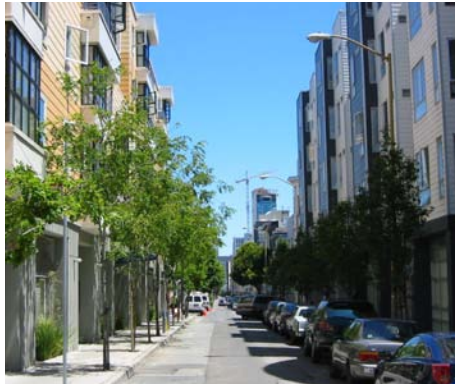
Figure 2. Example of 10th Street Mews, Natoma Street, South-of-Market in San Francisco. The right of way is just 35’, but still wide enough for sidewalks, one-way traffic and on-street parking.
