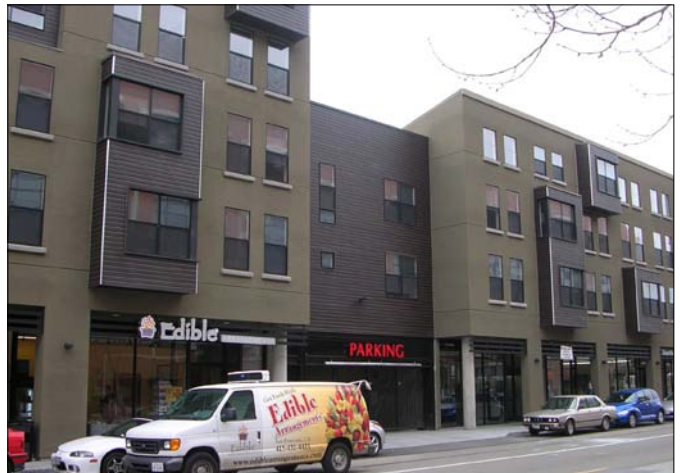
Figure 1: Vehicle access to the parking area is integrated into the massing of this mixed use building in building San Francisco. The parking is "wrapped" on all sides, with retail at ground level and residential uses above. The parking entry is recessed into a notch and kept narrow.
