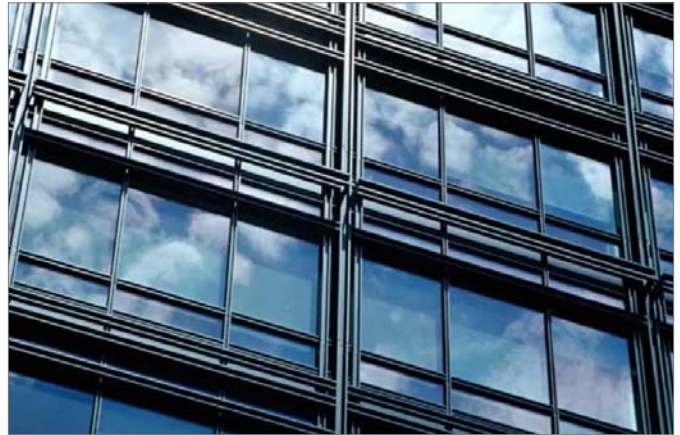
Figure 3. This office building at 560 Mission Street in San Francisco has a sophisticated system of projecting mullions and framing members, establishing an intricate dialogue between structure, skin and appendage.
