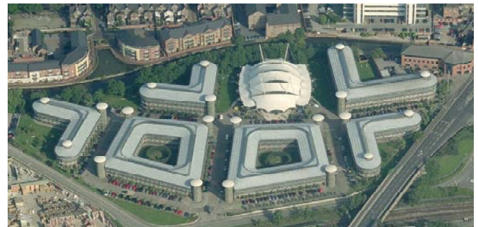
Figure 2. The commercial office buildings of the Inland Revenue Campus in Nottingham, England, utilizes narrow floorplates, allowing the buildings to passively regulate temperature and natural air ventilation whilst conserving energy.
