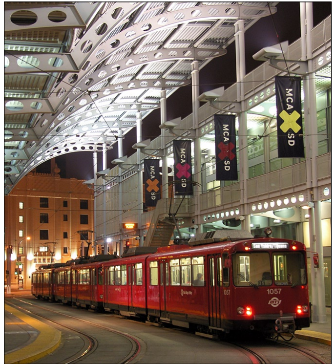
Figure 3.25. San Diego American Plaza Trolley Station integrates public light rail system into the privately developed 34-story highrise and the San Diego Museum of Contemporary Art. The museum is a focal point of the transit station.
