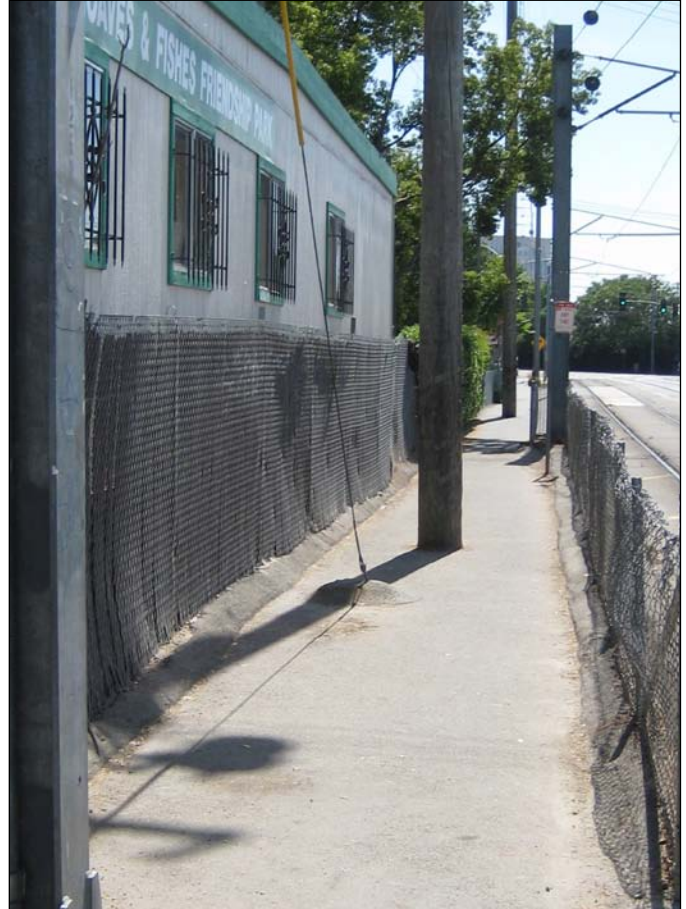
Figure 3.38. Many impairments are presented to the pedestrian on the east side of North 12th Street.
