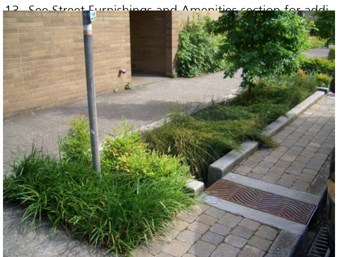
Urban stormwater management, in Amenity Zone, such as these planters and permeable pavement attenuate and treat stormwater flow.
