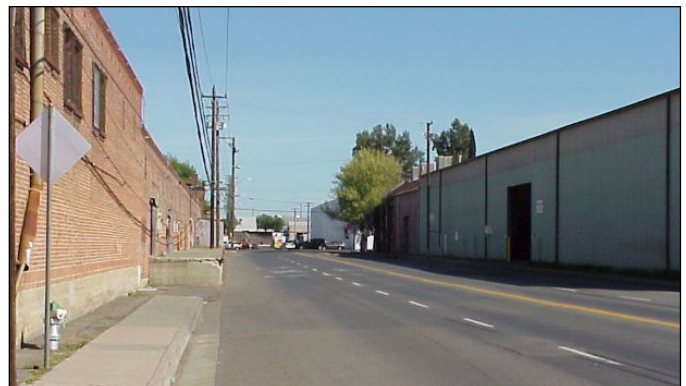
Figure 3.37. North B Street, east of Ahern, showing existing loading docks which may encroach into the public way. The brick facade of the General Produce building is within the North 16th Street Historic District.
