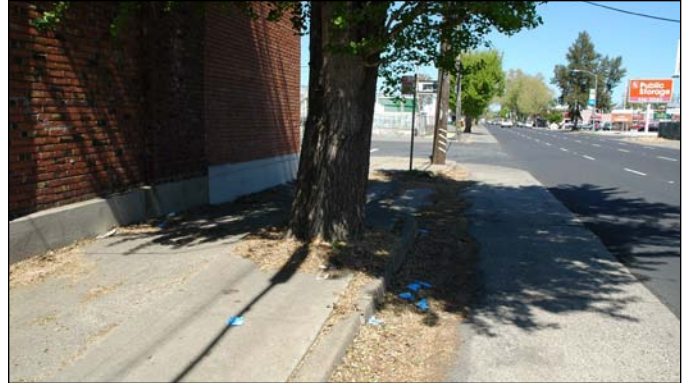
Figure 3.40. Sidewalks along North 16th Street have uneven surfaces and under-utilized laneways which could be converted to parking uses with the reconstruction of sidewalks.
