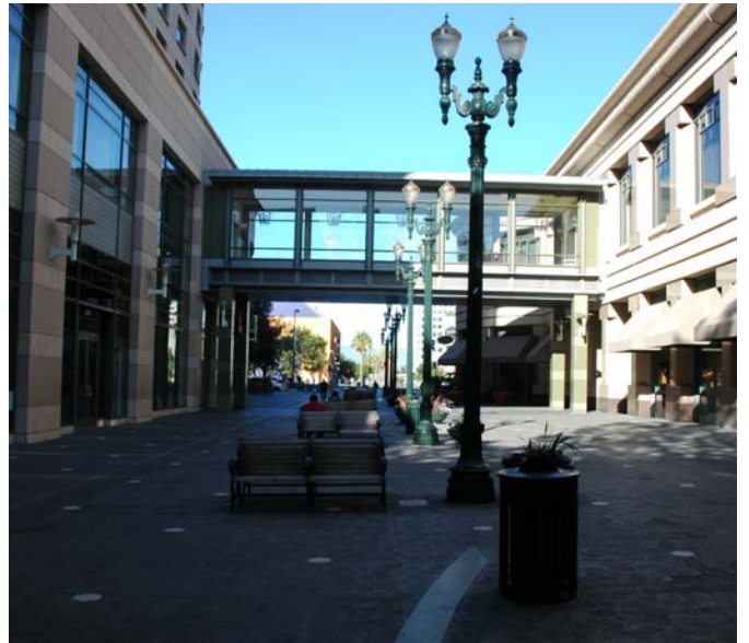
An example of an enclosed pedestrian bridge over a public plaza that has a high ratio of glass and fits into the architectural compositions of adjacent buildings.
