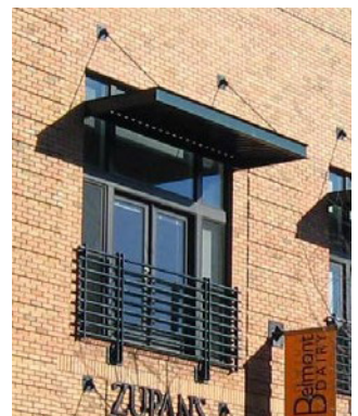
Figure 4-155. French balcony covering windows & operable doors
