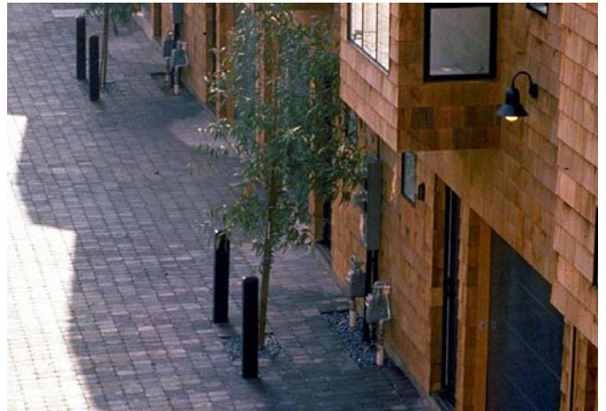
Figure 4-29. Utilities connections should be carefully located and integrated into the rhythm of the design
