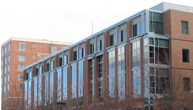
Figure 4-137. This university building in Cambridge, MA, has a repeating double window bay module which sets a rhythm across the façade, which is then interrupted by special conditions at the corner and above the entry.
