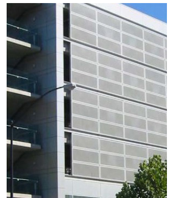
Figures 4-239 and 4-240. Parking structure at City Hall in San Jose, CA, uses horizontal metal louvers (left) and perforated metal panels (right) to control the glare produced by night lighting.
