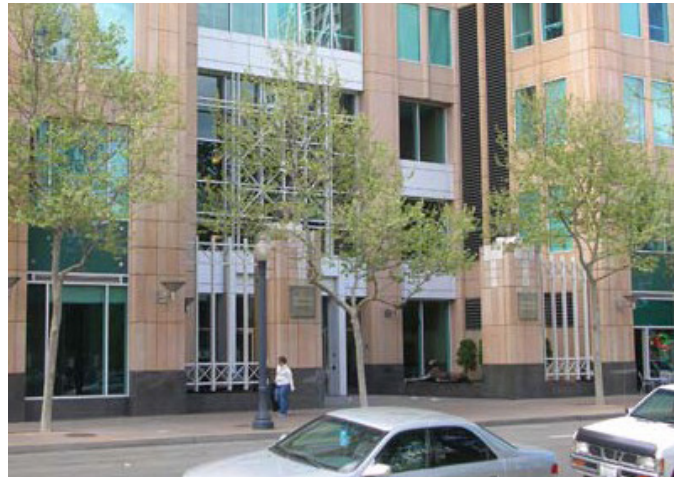
Figure 4-13. Public open space - forecourt in front of Park Plaza Tower, Sacramento.
