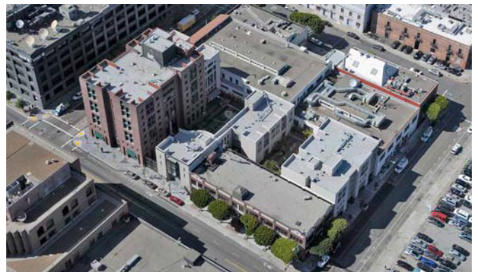
Figure 4-25: This apartment building development includes two building types in close proximity: mid-rise stacked flats (in red brick) and low-rise, wood frame residential building (cream colored).
