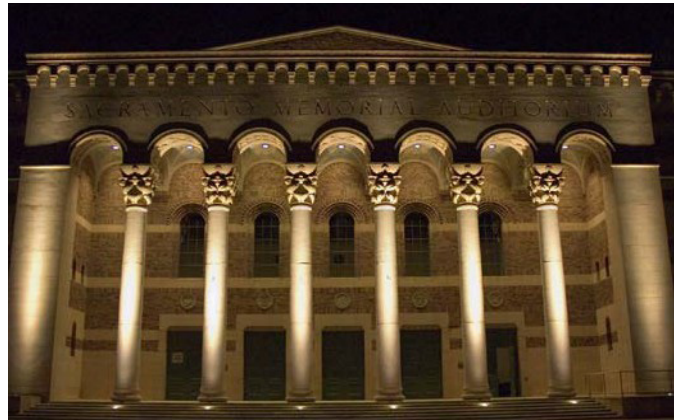
Figure 4-169. Exterior Lighting on Memorial Auditorium highlights the architectural features of the historic building.
