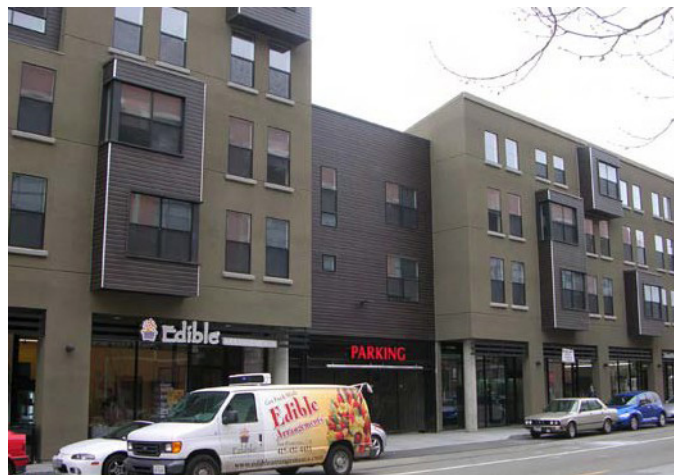
Figure 4-228. Vehicle access to the parking area is integrated into the massing of this mixed use building in building San Francisco. The parking is "wrapped" on all sides, with retail at ground level and residential uses above. The parking entry is recessed into a notch and kept narrow.
