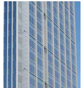
Figure 4-122. The facade of 621 capitol Mall has horizontal articulation every three floors, and a notch running vertically from top to bottom.
