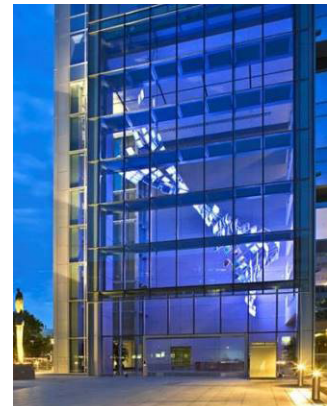
Figure 4-220. The LED sculpture "Rapids" dramatically activates the monumental entrance lobby and plaza approach at 621 Capitol Mall.
