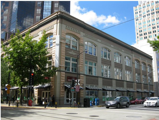
Figure 4-260. Hale Brothers & Company Building
