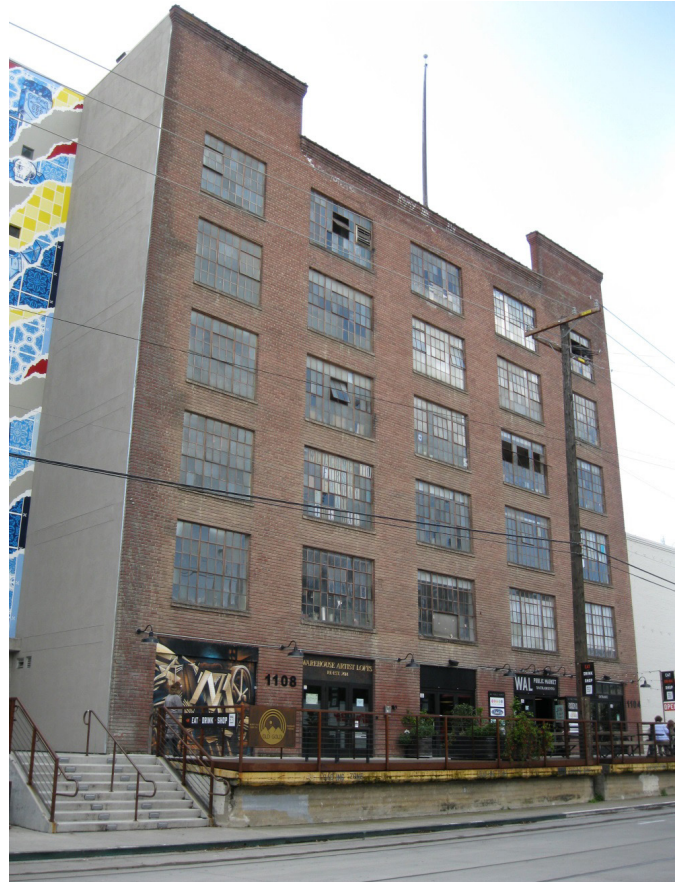
Figure 4-263. Sacramento Warehouse Company Building
