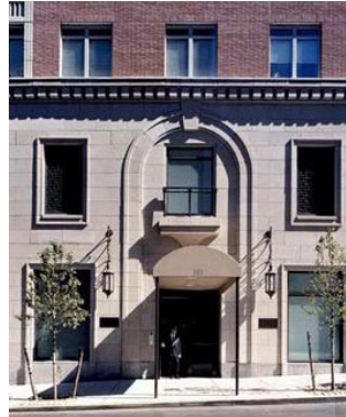
Figure 4-147. Entrance canopy to a residential apartment building on a downtown street.
