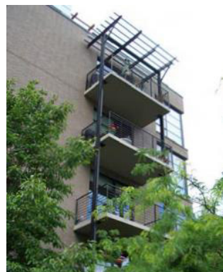
Figure 4-154. Stacked balconies on an apartment building
