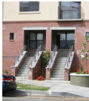
Figure 4-143. Entrances to individual units should orient to the street & be characterized by stoops, porches etc.
