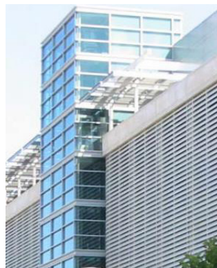
Figures 4-239 and 4-240. Parking structure at City Hall in San Jose, CA, uses horizontal metal louvers (left) and perforated metal panels (right) to control the glare produced by night lighting.
