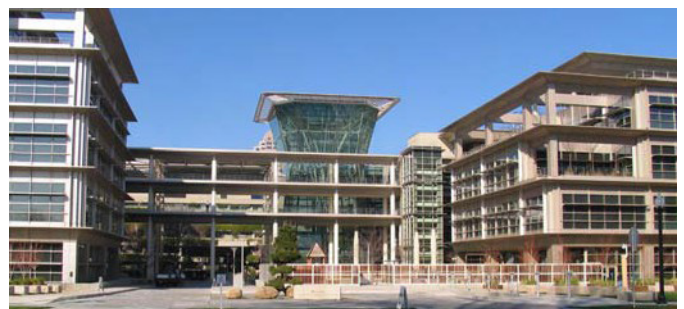
Figure 4-194. The LEED-certified CalPERS Building incorporates many sustainable design features that significantly impact the formal design of the building, including light shelves and abundant
