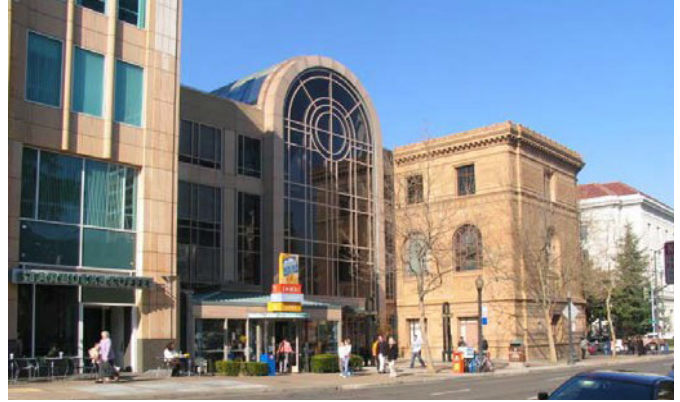
Figure 4-267. On Cesar Chavez Plaza, newer buildings mix with Sacramento's landmark civic buildings
