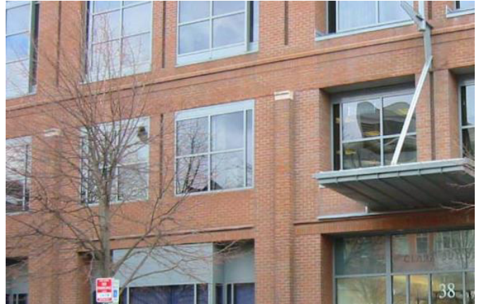
Figure 4-136. This building also combines curtain wall window systems with solid punched-opening walls. The wall is given a visual thickness by the varying placement of the glass line.
