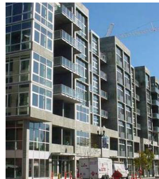
Figure 4-121 A wide street frontage is articulated with bay windows, projecting balconies, and recessed zones. The major massing articulations begin above the 2nd floor.
