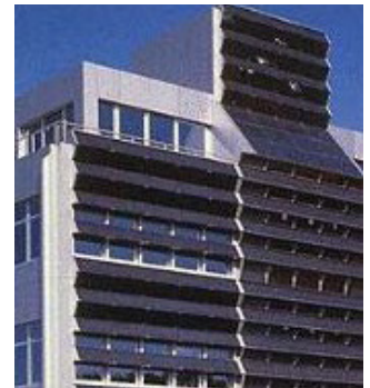
Figures 4-207 and 4-208. Building Integrate Photo Voltaic Panels. An integrated cladding element.
