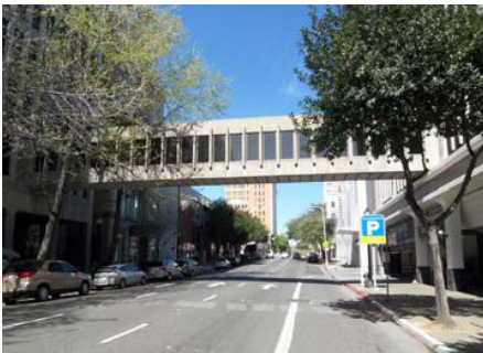
Figure 4-188. Pedestrian bridges over streets should be avoided as they remove pedestrian activity from the street.
