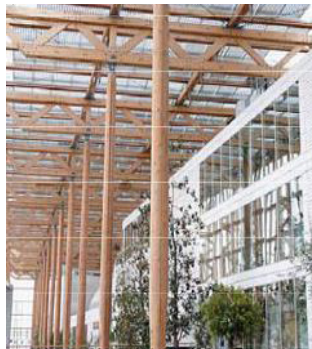
Figures 4-205 and 4-206. Photo Voltaic panel arrays, used to cover vast
