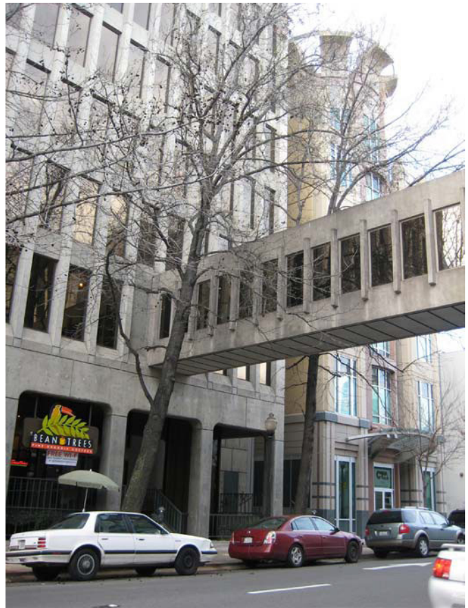
Figure 3-32. The pedestrian bridge at 10th and L St. blocks views and detracts from ground-floor pedestrian activity.
