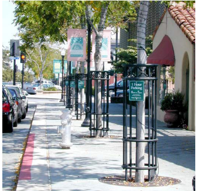
Figure 3-73. Tree grate with integrated tree guards in areas with high pedestrian use.
