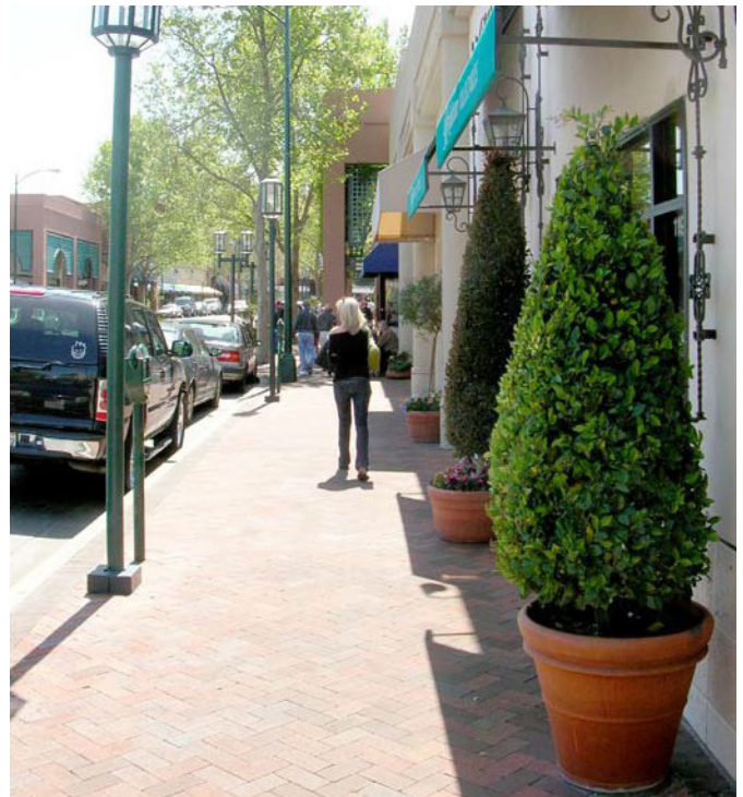
Figure 3-56. In cases where tree plantings are infeasible within the public amenity zone, planters within the frontage zone can provide a landscape element to the streetscape.
