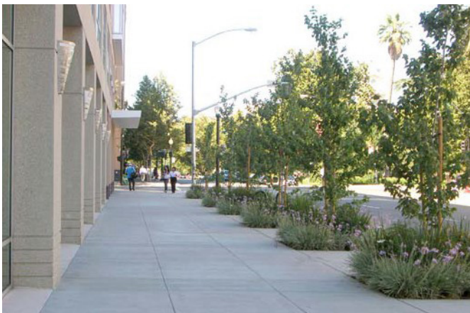
Figure 3-39. Sidewalk paving should be divided into a grid that fits the typical 16 foot wide sidewalk.
