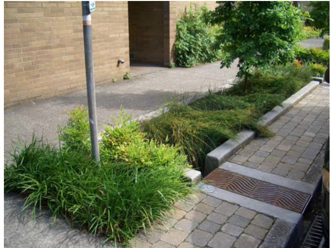
Figure 3-53. Urban storm-water management strategies such as these planters and permeable pavement attenuate and treat storm-water flow.
