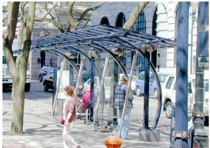
Figure 3-62. Attractive transit facilities, such as comfortable shelters with posted route information, encourage transit use.
