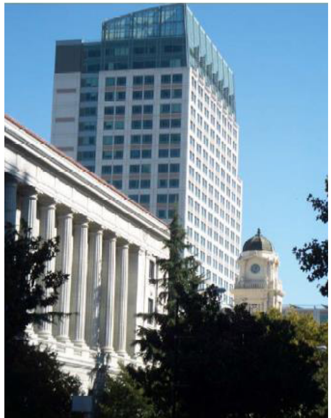
Figure 2-17. Sensitive selection of colors and materials on new tower blends old and new into harmonious whole.
