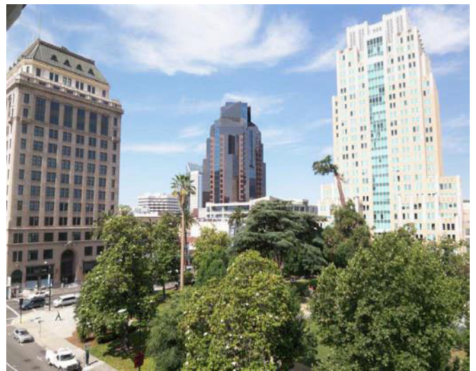
Figure 2-6. Building on left represents traditional historic form with vertical ribbons of punched window groupings, strong base, middle and a distinctive roof top. The street wall is well defined with a hierarchy of horizontal comicing utilizing local terracotta exterior details and cladding. High rise tower in center exhibits “contrasting” architectural elements to interject visual tension to skyline. High-rise tower at right side employs creative re-interpretation of “punched” fenestration groupings. The building massing, distinctive roof top element and exterior coloration harmonize with the neighboring historic structures.
