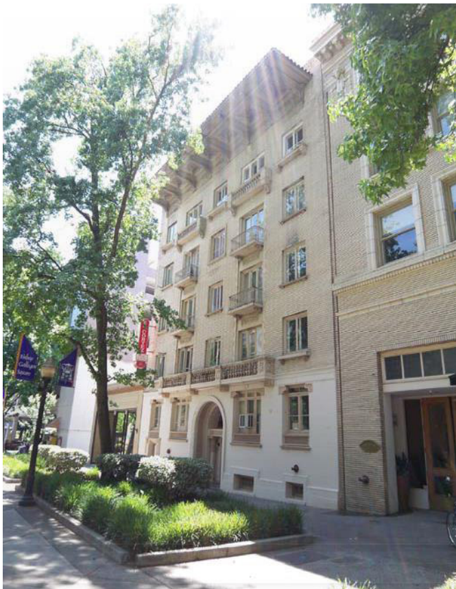
Figure 2-16. Traditional architecture unites base, middle, and distinctive top section with vertically oriented punched openings.
