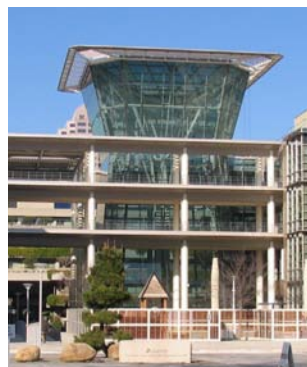
Figure 4. The CalPERS Building, Sacramento, CA. The building regulates air ventilation by channelling warm air up and out through the glass atrium.
