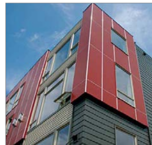
Figure 3. Exterior wood panels
