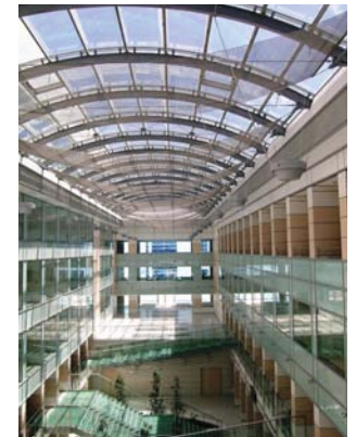
Figures 3 and 4. Internal sky-lit atria, allowing daylight light to penetrate to a maximum amount of internal space, at all floors
