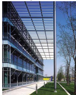
Figure 1. Giant canopy applied to a commercial office building, Chiswick Park, London, UK.
