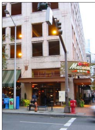
Figure 6. Parking structure in downtown Portland, Oregon, where the facades designs emulate the character of the neighborhood.
