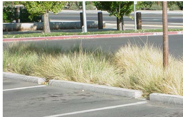
Figure 2. Sustainable stormwater management: parking area drains to bioswale rain-garden
