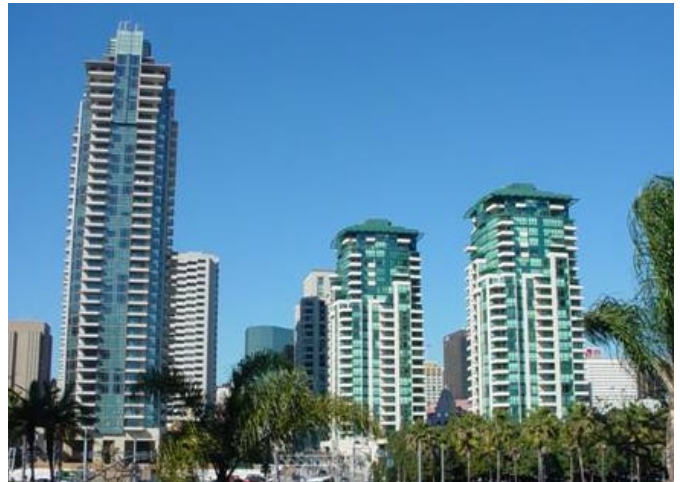
Figure 2: High-rise residential buildings- shown here in downtown San Diego- typically have minimal ability to accommodate stepback recommendations, due to the requirements for residential units to "stack" in a repetitive fashion. Massing articulations are often found in balcony and terrace configurations.
