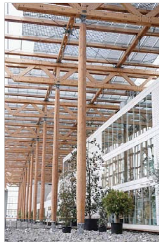
Figures 3 and 4. Photo Voltaic panel arrays, used to cover vast areas over a building roof (above) or mounted on a giant trellis (below), where they also function as a sunshading element.
