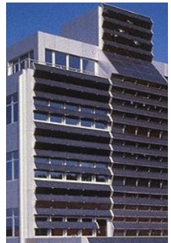
Figures 5 and 6. Building Integrate Photo Voltaic Panels, used as an integrated cladding element as well as for sunshading.
