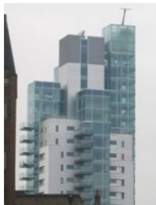
Figures 4 and 5: Two views of a new 25-story high-rise residential tower in London. The floorplates have no stepbacks until the top eight stories, where the "bundled" vertical masses successively end, creating terraces for the upper floors.
