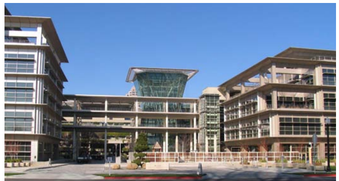
Figure 3. The LEED-certified CalPERS Building incorporates many sustainable design features that significantly impact the formal design of the building, including light shelves and abundant daylighting.
