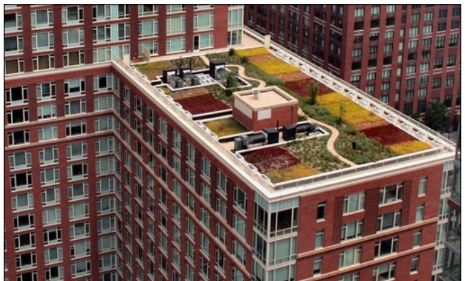
Figures 5. Green roof on an urban high-rise residential building.
