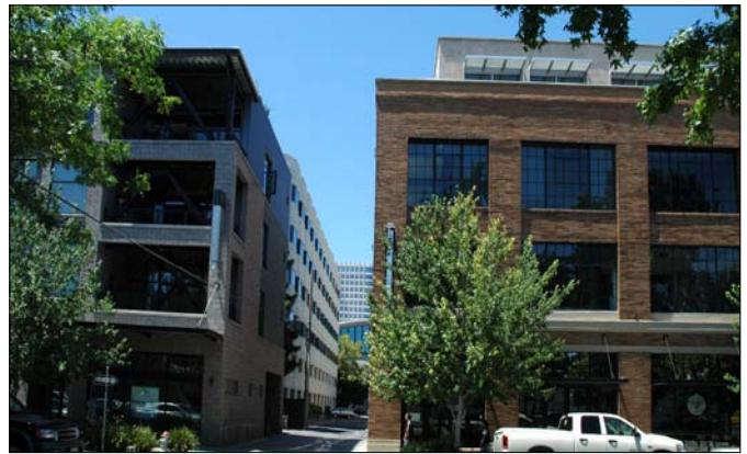
Figure 1. The new building on the left maintains the scale and proportion of mass and fenestration in keeping with the historic building on the right.
