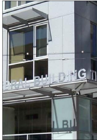
Figure 1. New block letter signage wrapping the corner of the Cathedral Building.
