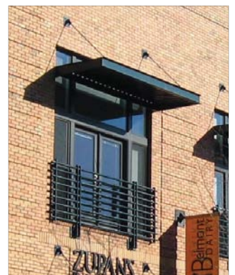
Figure 5. French balcony covering windows & operable doors
