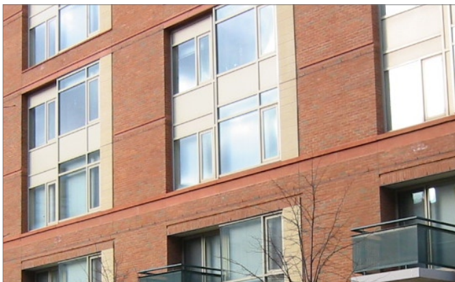
Figure 4. This project inserts a curtain wall system within a punched opening. The red brick wall turns to reveal the wall's thickness, and the curtain wall is placed at varying depths within the apparent thickness of the brick wall opening.
