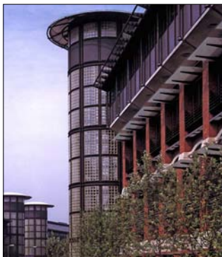
Figure 3. Inland Revenue Center, UK. The building passively regulates temperature and natural air ventilation, allowing warm air to exhaust through the stairwells.
