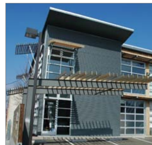
Figure 5. Industrial metal siding
