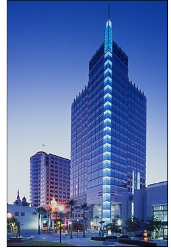
Figure 5. The Esquire Building's lighting design includes a dramatic illuminated corner.
