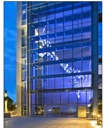
Figure 10. The LED sculpture "Rapids" dramatically activates the monumental entrance lobby and plaza approach at 621 Capitol Mall.
