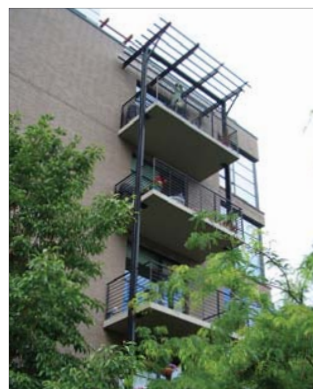
Figure 4. Stacked balconies on an apartment building
