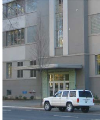
Figure 1. Vertical elements and canopy mark the entrance to the Department of Transportation building, Sacramento
