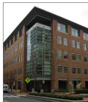
Figures 7 & 8. Different materials and colors should be separated with a change in plane.
