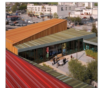
Figure 6. Metal wall and roof panels
