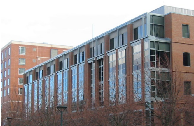
Figure 2. This university building in Cambridge, MA, has a repeating double window bay module which sets a rhythm across the facade, which is then interrupted by special conditions at the corner and above the entry.
