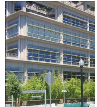
Figure 6. The CalPERS building, with horizontal sunshades and light shelves.
