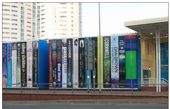
Figure 3: The temporary construction screening for the new City of Cardiff (Wales) Library depicts giant book spines.
