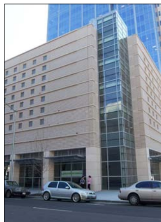
Figure 7. Parking structure at 621 Capitol Mall, with mixed uses lining the street-level spaces.
