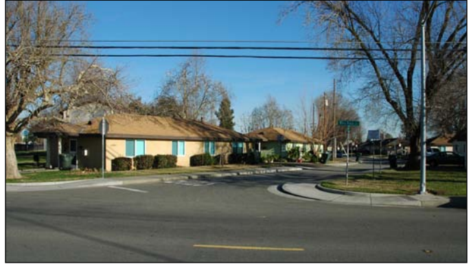
Figure 3.43. The existing low-density Twin Rivers Community will see future redevelopment that replaces the single family and two story townhomes with aggregated units and additional common park space centered on a new promenade street.
