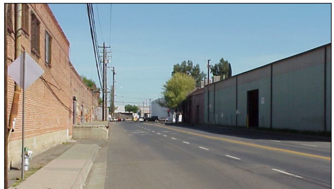
Figure 3.37. North B Street, east of Ahern, showing existing loading docks which may encroach into the public way. The brick facade of the General Produce building is within the North 16th Street Historic District.
