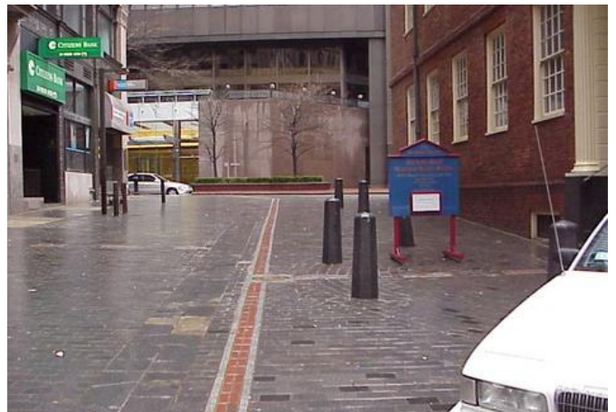
The Freedom Trail in Boston is demarcated in the paving with a line of brick pavers. A similar paving system can be implemented to denote routes for Park Links and River Streets
