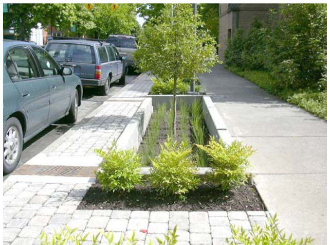
Permeable pavement and rain gardens provide stormwater management benefits (Portland, OR).
