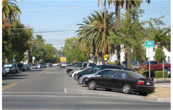
Back-in angled parking provides for convenient loading and unloading and is safer for bicyclists (28th St. between R St. and U St.)
