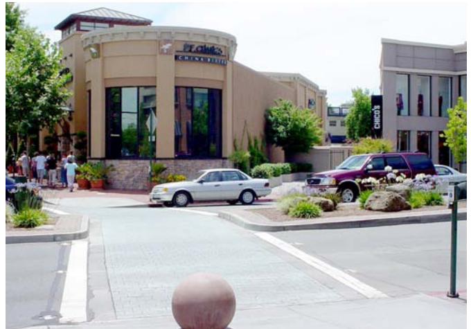
Special paving treatments and pedestrian-activated crossing lights alert drivers to the presence of pedestrians.
