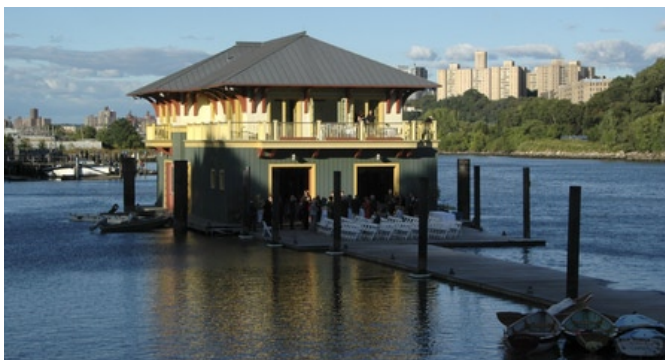
Figure 3.7 Boathouse on the Harlem River, New York. Floating facilities bridged from the levee crown can offer paddle-craft opportunities for exploring the river.
