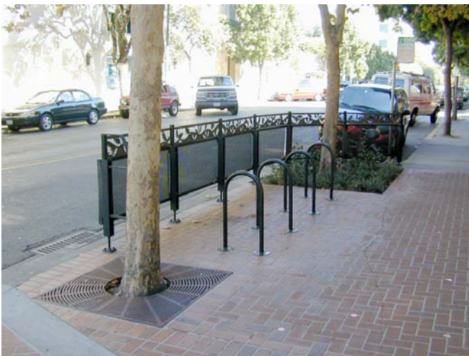
Expanded sidewalk with bicycle parking.
