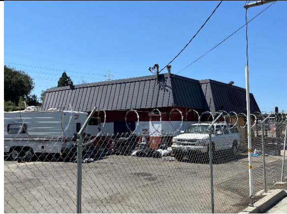
Figure 2. East facade, view southwest.
