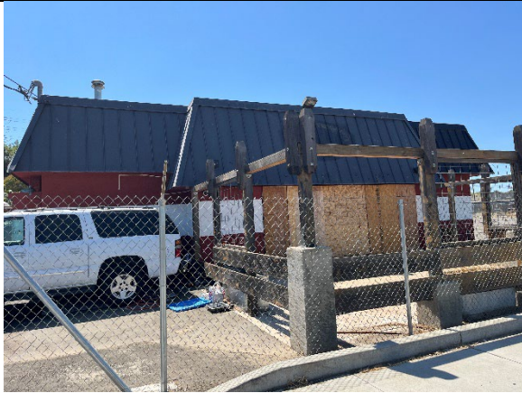
Figure 1. North facade, view southwest.
