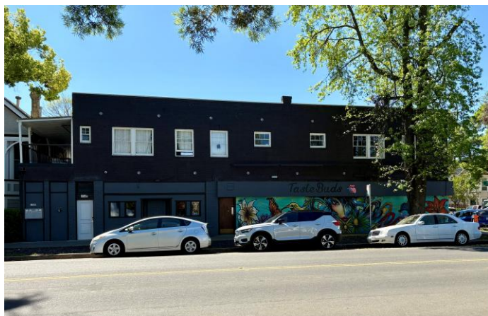
Figure 6: North façade, view south
