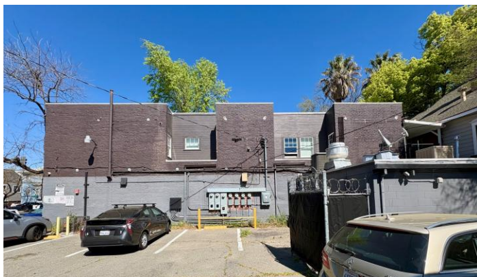
Figure 4: South façade, view north
