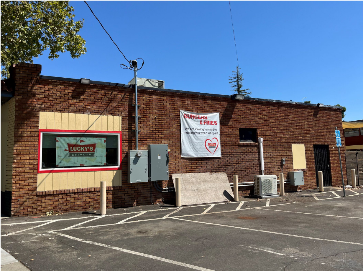
Figure 1. South facade, view northeast.
