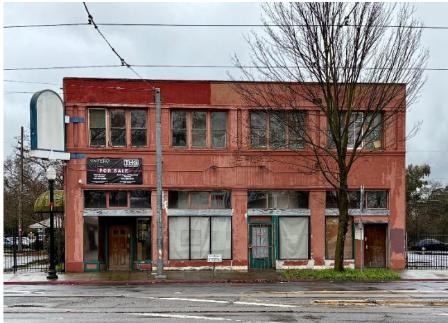
Figure 1. Southeast façade, view northwest.
