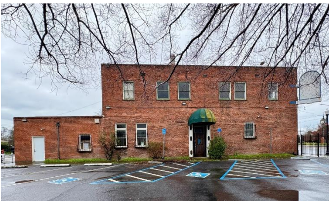
Figure 3. Southwest façade, view northeast
