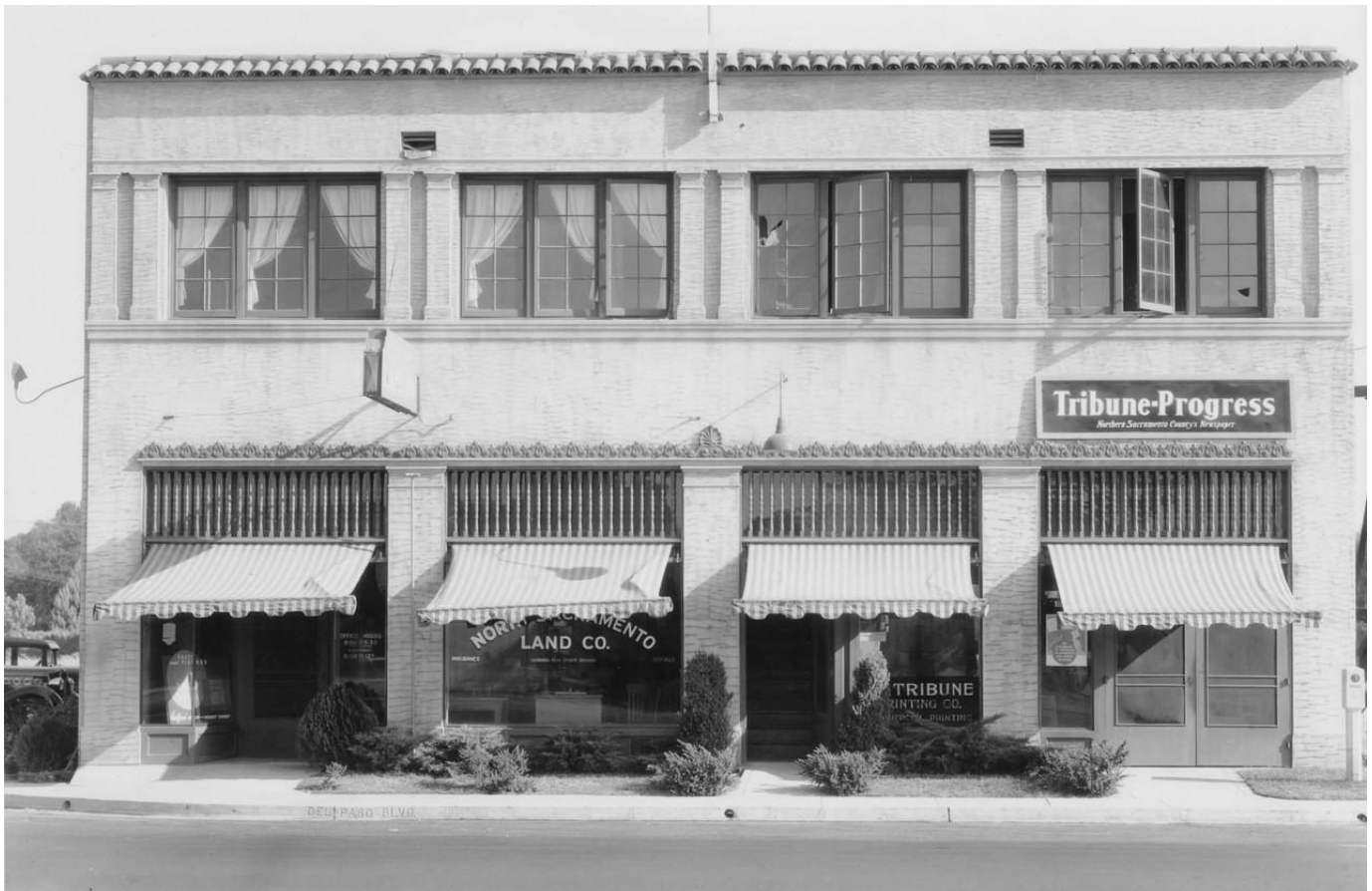
Figure 8: 1454 Del Paso Boulevard. Source: Center for Sacramento History, Facebook post January 7, 2025.
