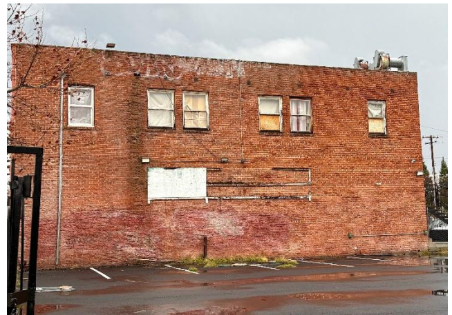
Figure 2. Northeast façade, view southwest
