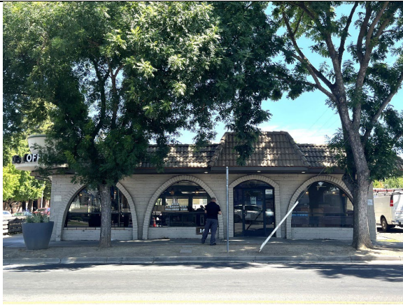
Figure 1. Northwest facade, view southeast.
