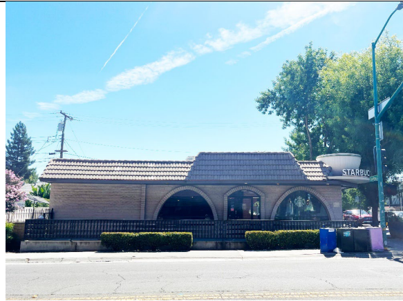
Figure 2. Northeast facade, view southeast.
