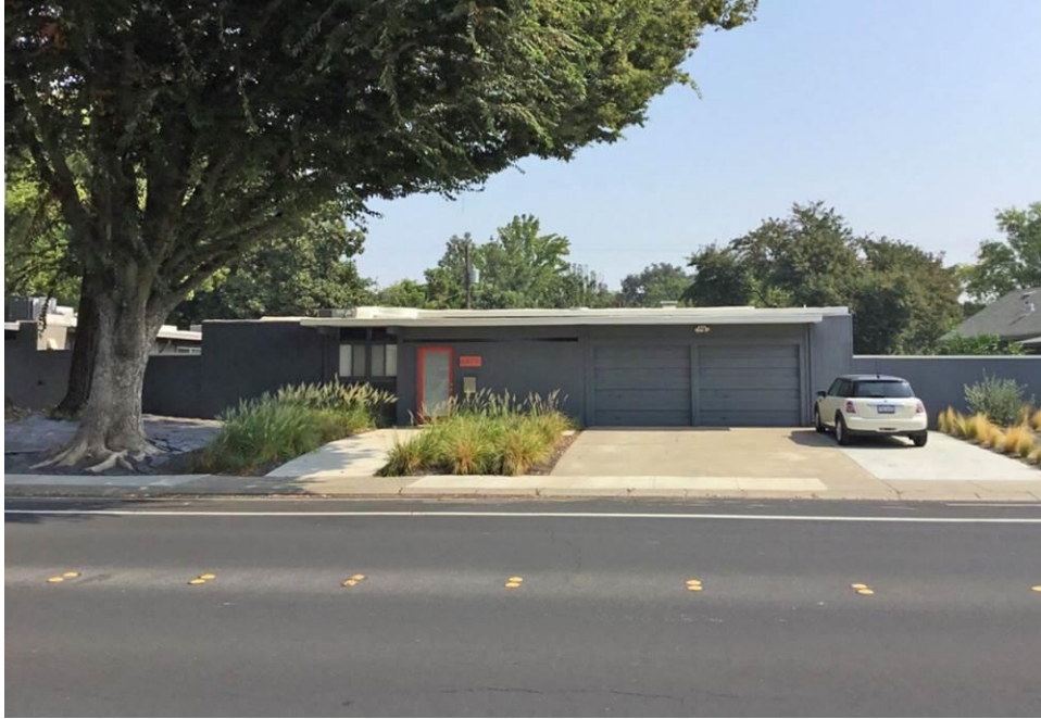
Photograph 9. 6473 South Land Park Drive, camera facing northeast September 2, 2017
