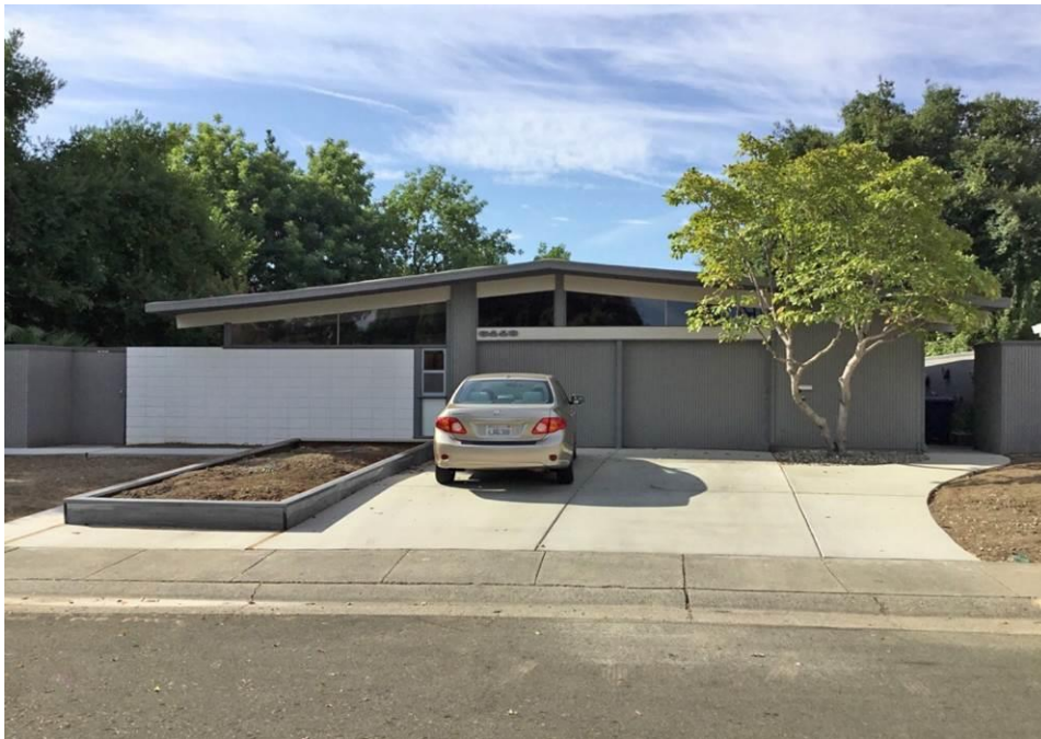
Photograph 15. 6448 Oakridge Way, camera facing south September 17, 2017
