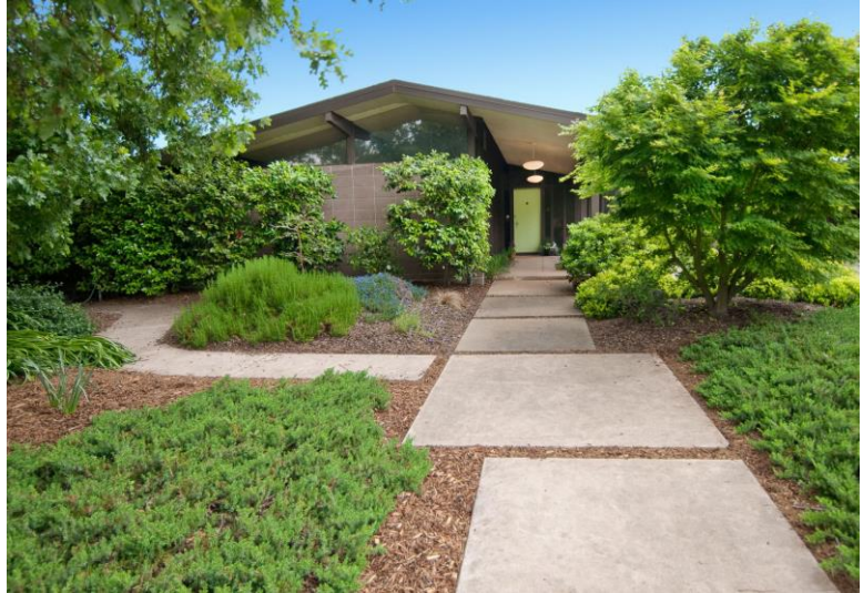
Former Stecher Residence, 6170 Wycliffe Way Architect: Carter Sparks and Donald Thaden, 1960 Source: SacMod, 2010
