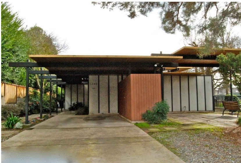
1240 Kaylar Drive Architect: Carter Sparks and Donald Thaden, 1957 Source: SacMod, 2017
