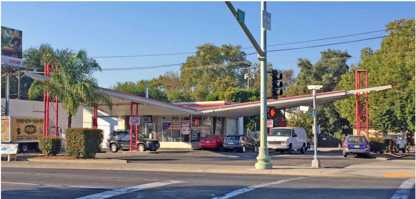
2025 Broadway Architect: Clarence Reinhardt, 1960 Source: SacMod, 2017
