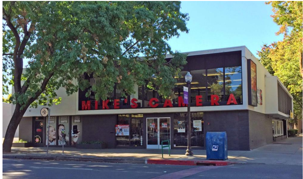
Figure 13. Former Fort Sutter Savings & Loan Association
