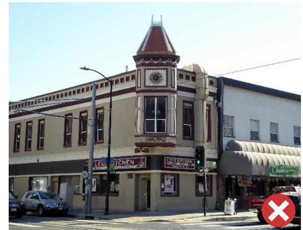
Figure 185. Many of the historic exterior features of this contributing building have been preserved and maintained; however, the windows and front facade have been partially covered by a ventilation duct.
