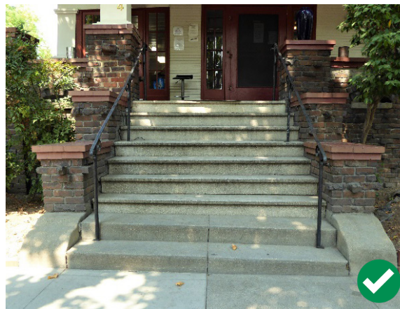
Figure 278. Wood, brick, and terrazzo are common materials used in historic architectural features in the historic district.
