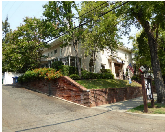
Figure 270. The former Charles McClatchy residence at 2112 22 nd Street, now the McClatchy Library. Many houses in the district, especially those planted on the “ridge” that gives the Poverty Ridge Historic District its name, have sloped lawns and low masonry retaining walls.
