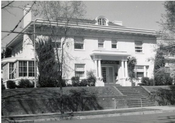
Figure 275. The McClatchy Library, formerly the Charles McClatchy house (1951). Source: Center for Sacramento History, Frank Christy Collection, 1998/722/1366.
