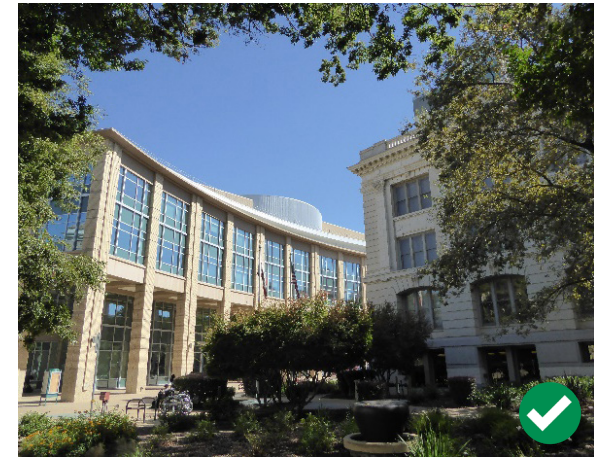
Figure 265. The addition to City Hall incorporates materials, height, scale, and a generous setback that are compatible with the historic building and maintain its primacy in the wider streetscape.
