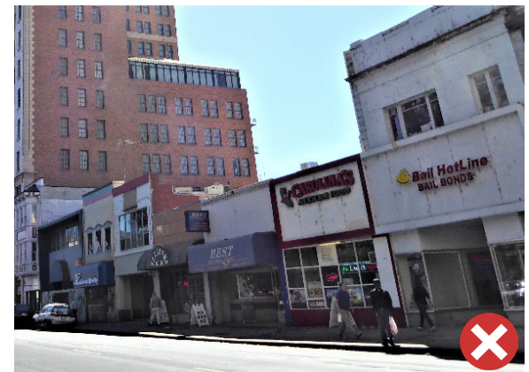
Figure 264. The historic facades, exterior materials, windows, and entries of several buildings on J Street have been covered with incompatible non-historic cladding and additions.
