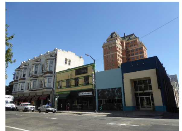
Figure 256. The district contains commercial buildings that display a wide variety of architectural styles and forms, such as these buildings on 9 th Street.
