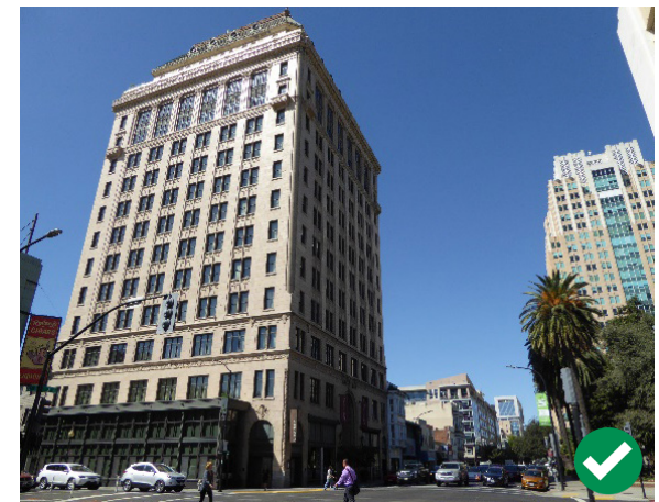
Figure 266. The California-Western States Life Insurance Building at 926 J Street is a visual focal point of the district.
