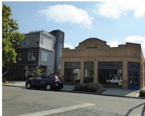
Figure 231. A One-Part Commercial Block building with a Mission-style parapet sits next to an infill housing development.
