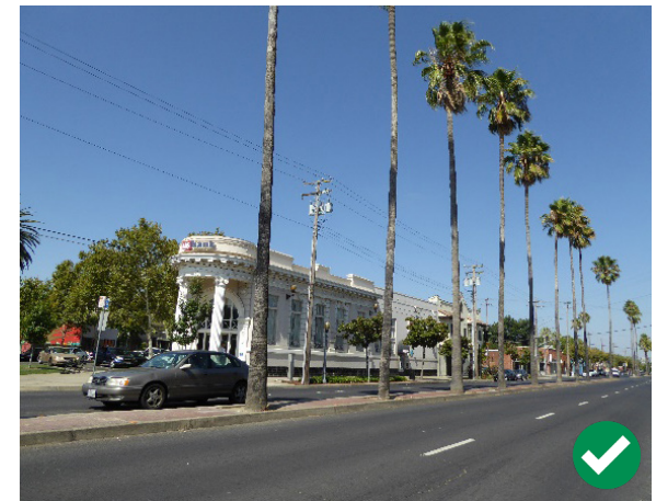
Figure 240. The regular rows of palms in the medians and diagonal alignment of Broadway are a character-defining features of the district.
