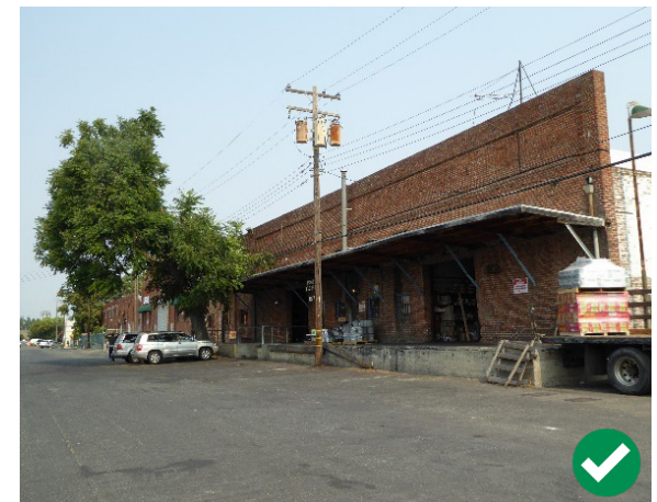
Figure 227. Historic awnings on contributing buildings may serve as an inspiration for the addition or design of compatible new awnings.
