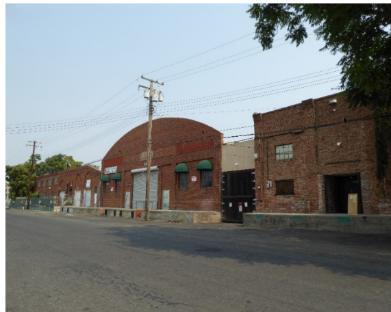
Figure 218. A row of one-story brick warehouses with raised concrete loading docks on North C Street, once part of the Triangle Produce Company.
