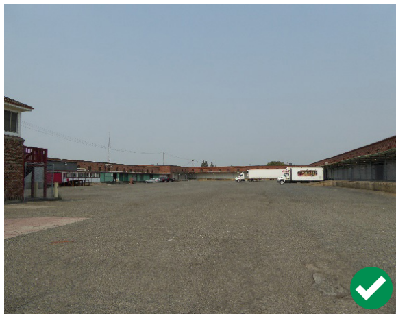
Figure 225. Open areas, such as the courtyard in this U-shaped produce distribution building, reflect their historic use as spaces for vehicle maneuvering.
