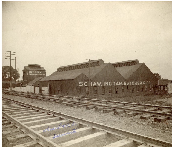
Figure 221. The Schaw, Ingram, Batcher & Co pipeworks situated along a spur of the Southern Pacific Railroad tracks (ca. 1900). Source: Center for Sacramento History, Frank Christy Collection, 1998/722/0299.
