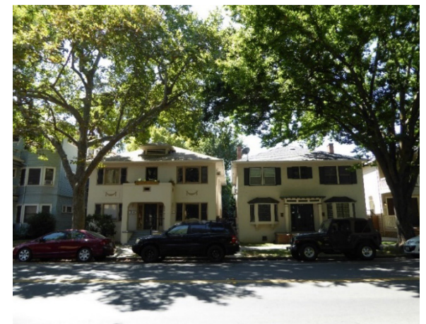
Figure 191. A few two-story apartment buildings sit side-by-side on G Street.
