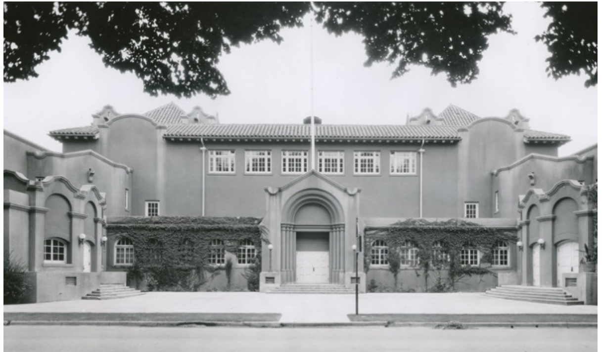
Figure 192. The Washington School at 18 th and E Streets (date unknown) prior to demolition. Source: California History Room, California State Library, Sacramento, California.
