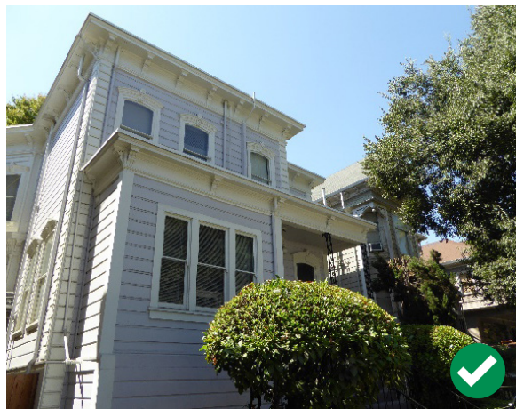
Figure 160. Contributing buildings on Q Street are predominately vertically massed.
