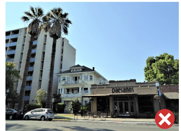
Figure 147. The height, massing, and materials of the building on the left are incompatible with the historic buildings on the right.
