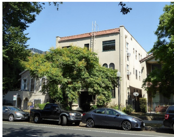
Figure 138. A mix of apartment buildings, some dating to the period of significance, are interspersed throughout the district.
