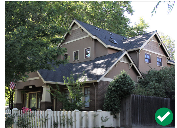
Figure 19. The rooftop addition on this house has been setback from the front facade.
