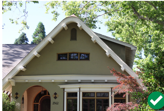
Figure 21. The new dormer on the right is compatible with the design of the original building.
