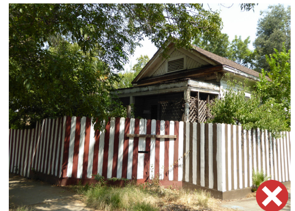
Figure 45. The height and opaque quality of this fence prevents views of the building's primary façade from the public right-of-way, as well as views of the street by the building occupants.
