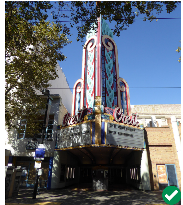
Figure 49. The original marquee of the Crest Theater is a good example of a preserved and restored historic lighting feature that is unique to its property type.
