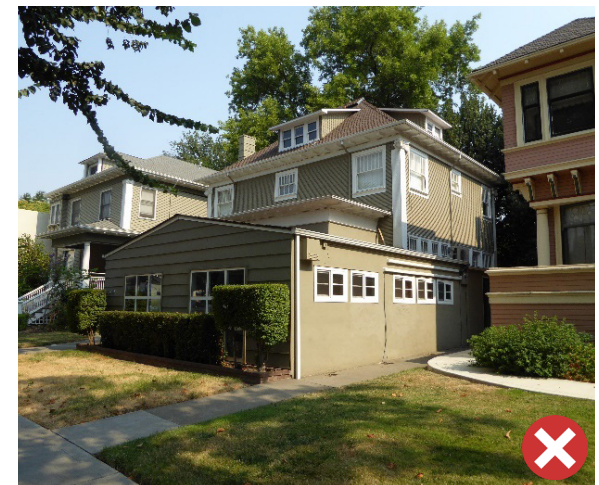
Figure 20. This addition has been added over the building's primary, street-facing facade and porch.
