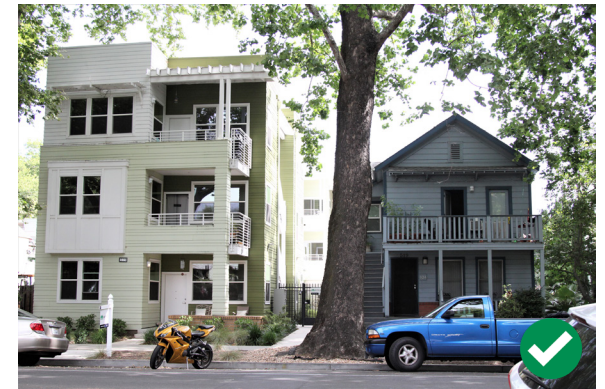
Figure 39. The horizontal window and opening datum lines of the infill on the left are aligned with those of the contributing building on the right.
