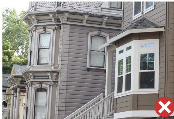
Figure 38. The use of vinyl frame windows with false divided lights are not compatible with the wood frame windows of the contributing building on the left.
