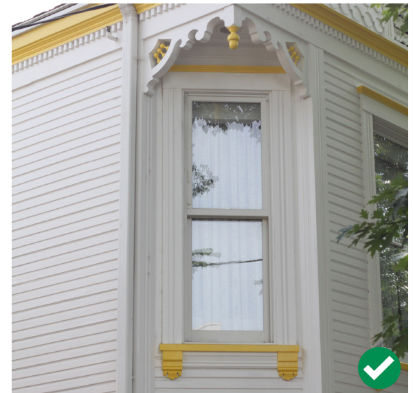
Figure 14. New double-hung windows have been installed on this house.
