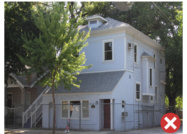
Figure 13. The porch and primary façade of this house have been covered by a later addition.
