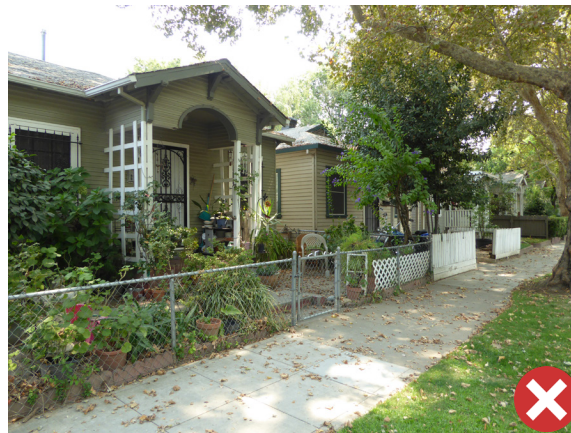
Figure 44. The scale of this fence is appropriate to the scale of the house; however, the use of chain link is not compatible with the predominately wood materials of the house and overall historic district.
