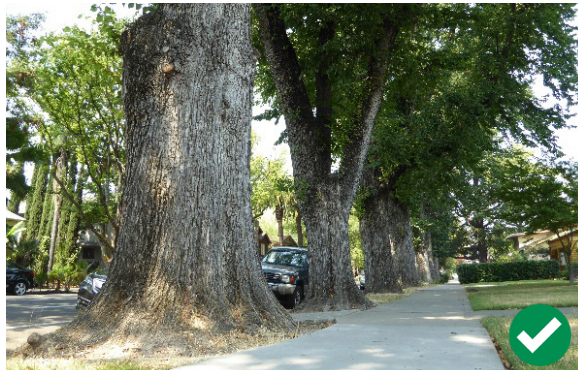
Figure 55. Parking strips planted with rows of mature street trees are a character-defining feature of many of Sacramento's historic districts.
