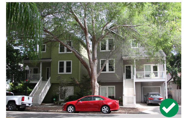
Figure 40. The proportions, depth, and materiality of the window and door openings of these infill buildings reflect those of many contributing buildings found throughout Sacramento's historic districts.
