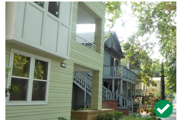
Figure 36. The materials of the new infill on the left echo the horizontal wood siding and features on the adjacent contributing building.
