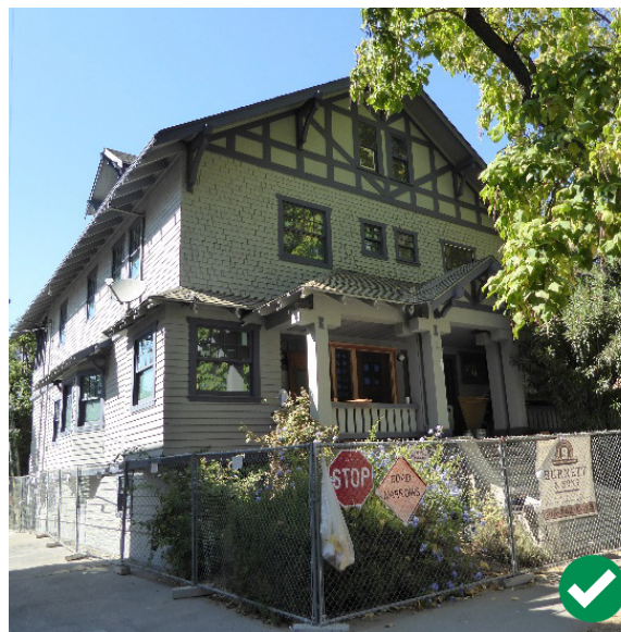
Figure 10. The window and door frames of this house have been replaced with new wood frames that match the original.
