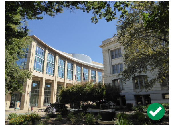
Figure 35. The City Hall extension features a contemporary design that respects and enhances the character of the surrounding historic district.
