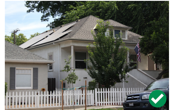
Figure 15. The solar panels and attic vents on the roof of this house are appropriately mounted so that they have a low profile and are minimally visible from the street.
