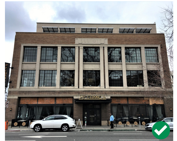
Figure 18. This rooftop addition does not detract from the character of the historic building, because it is setback from the primary facades.
