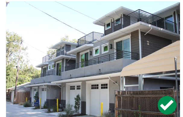
Figure 62. The taller massing of these three-story alley infill buildings has been stepped back from the alley face.
