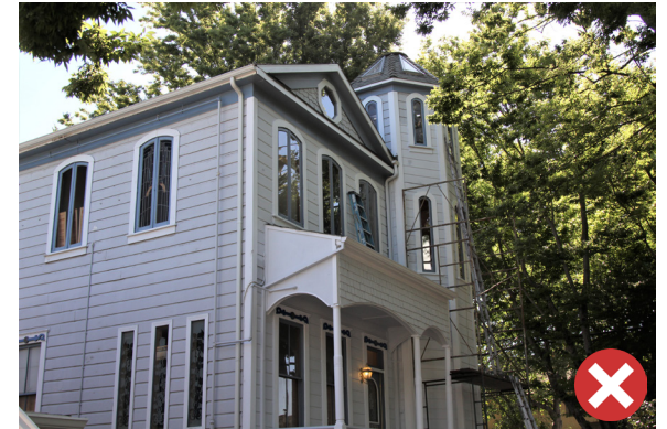
Figure 12. A new turret, porch, and window openings have been added to this house.
