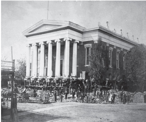
Figure 3. Sacramento's second county courthouse being raised (ca. 1870). Source: Center for Sacramento History, Sacramento Bee Collection, 1983/001/SBPM02400.
