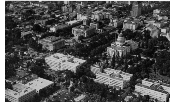
Figure 103. Aerial view of Sacramento, showing the Capitol Extension Group to the west of Capitol Park and the complete Business and Professional Building, Department of Motor Vehicles Building, and Department of Public Works Building along N Street (1940). Source: Special Collections of the Sacramento Public Library.
