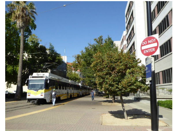
Figure 99. The tracks of the Sacramento Regional Transit light rail and several parking lots line O Street to the south of the district.
