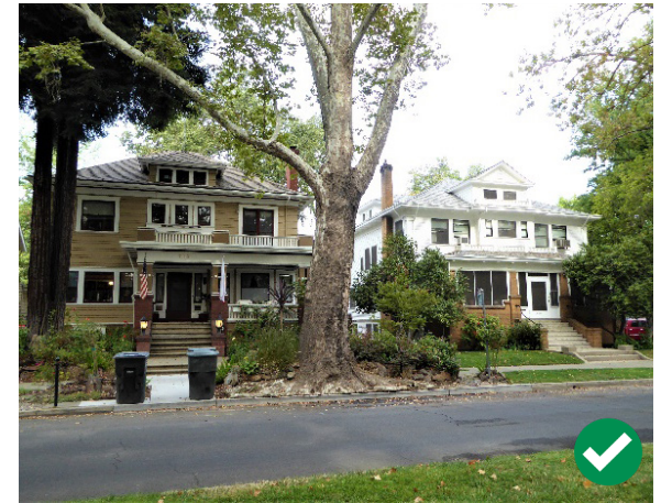
Figure 65. Large, Classic Box style houses with box-like massing are common on many blocks in the district.
