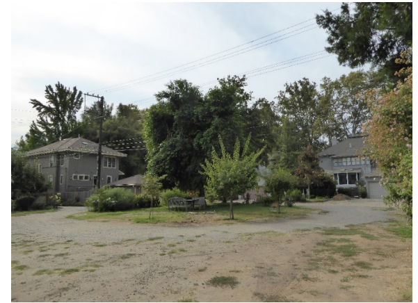
Figure 56. The alley parks that were part of the Wright and Kimbrough planned subdivision survive on three blocks behind the houses on 21 st Street between G and H streets.
