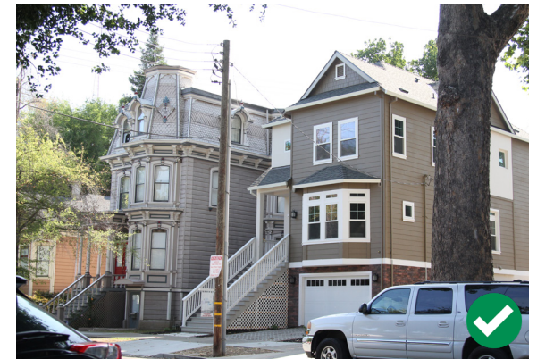
Figure 50. The majority of contributing buildings in the district exhibit narrow, vertical massing.
