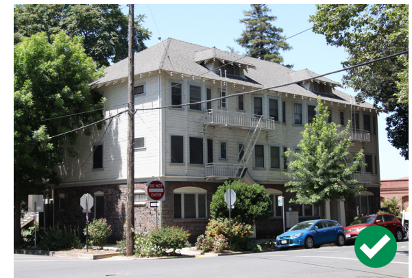
Figure 51. Alkali Flat West displays a mix of historic single- and multi-family housing types that can be used as design inspiration for new infill.
