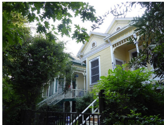
Figure 23. A row of nearly identical Queen Anne houses on 11 th Street in the Alkali Flat North Historic District.
