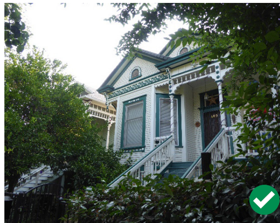
Figure 39. The ornate houses at 405-415 11 th Street create a particularly cohesive grouping of houses that should be carefully preserved.
