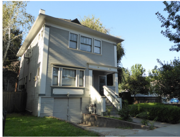
Figure 10. A Classic Box house beside the former Western Pacific Railroad tracks that form the historic district's western boundary.
