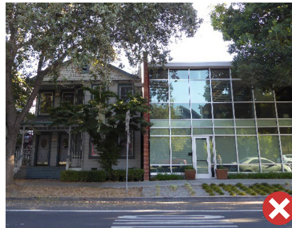
Figure 19. The new office building does not have an appropriate site setback from the historic building.
